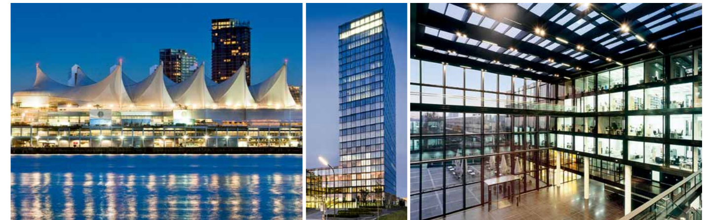
Thanks to lighting and building technology from Siemens, the Vancouver Convention Center (left) and the headquarters of Germany's Süddeutscher newspaper meet the highest efficiency standards.
