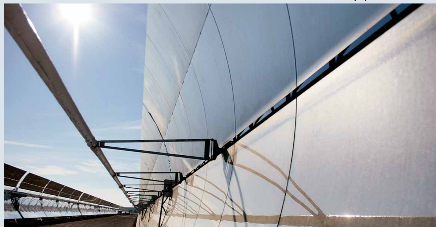
Solar thermal power plants with parabolic mirrors that track the sun are an established technology for the production of electricity. Below: Siemens' Lebrija 1 plant near Seville.
