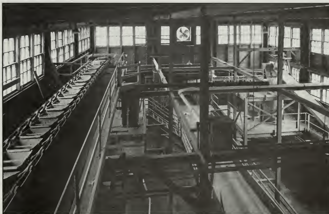
Photo 83. Harbison-Walker, interior view with bucket line feeding molding machine on left. Photo by Jet Lowe.
