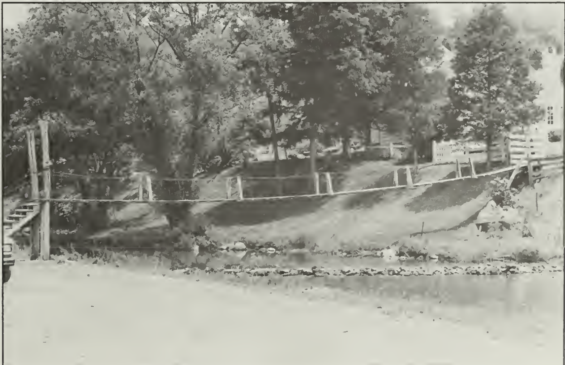
Photo 45. Swinging bridge over Stone Creek.
