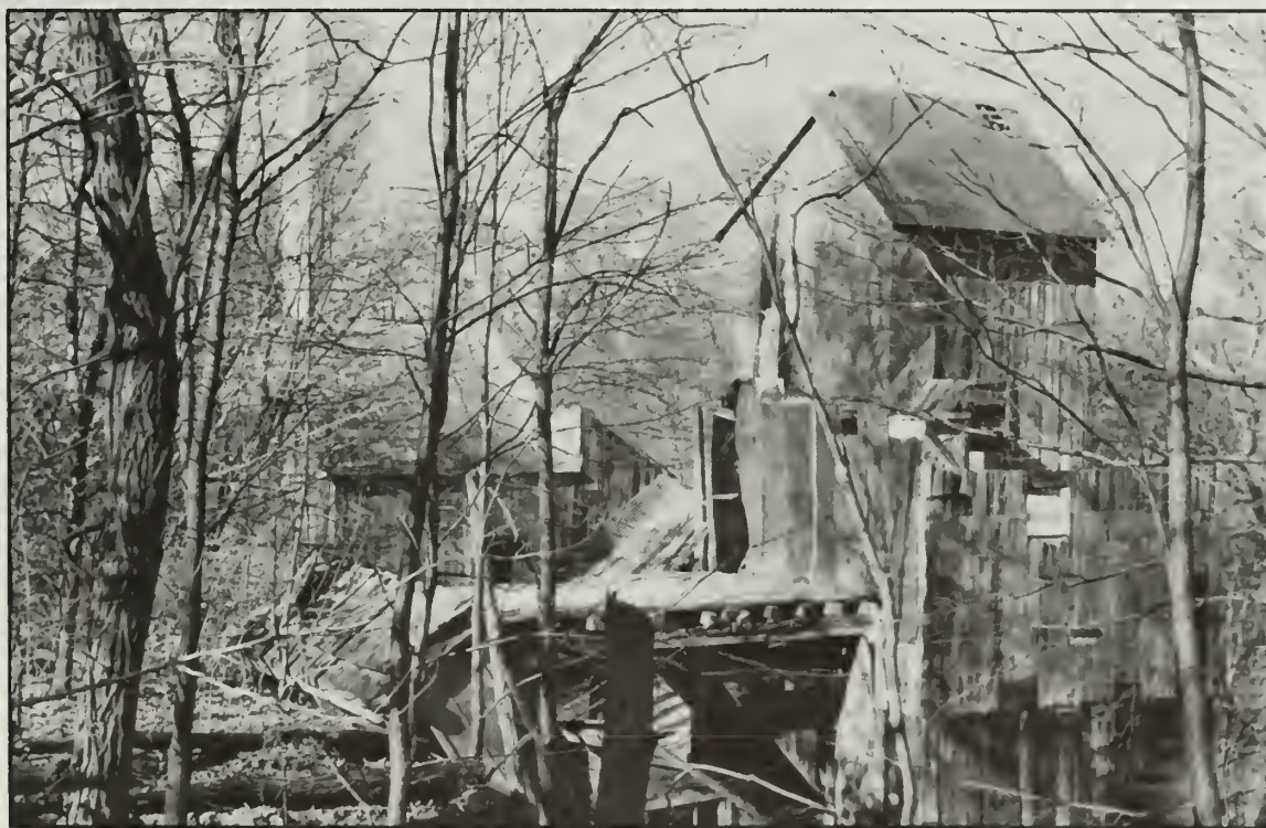
Photo 70. Hatfield and Phillips Fire Clay Company.
