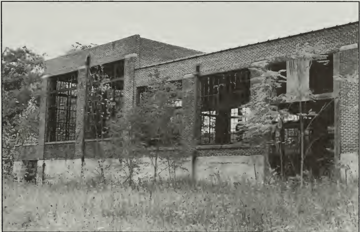
Photo 24. Boyle Ice Plant.
