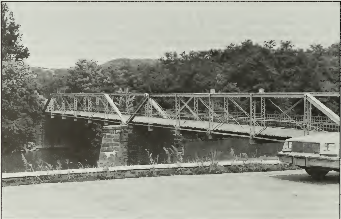
Photo 44. State Reformatory bridge to Cypress Island.
