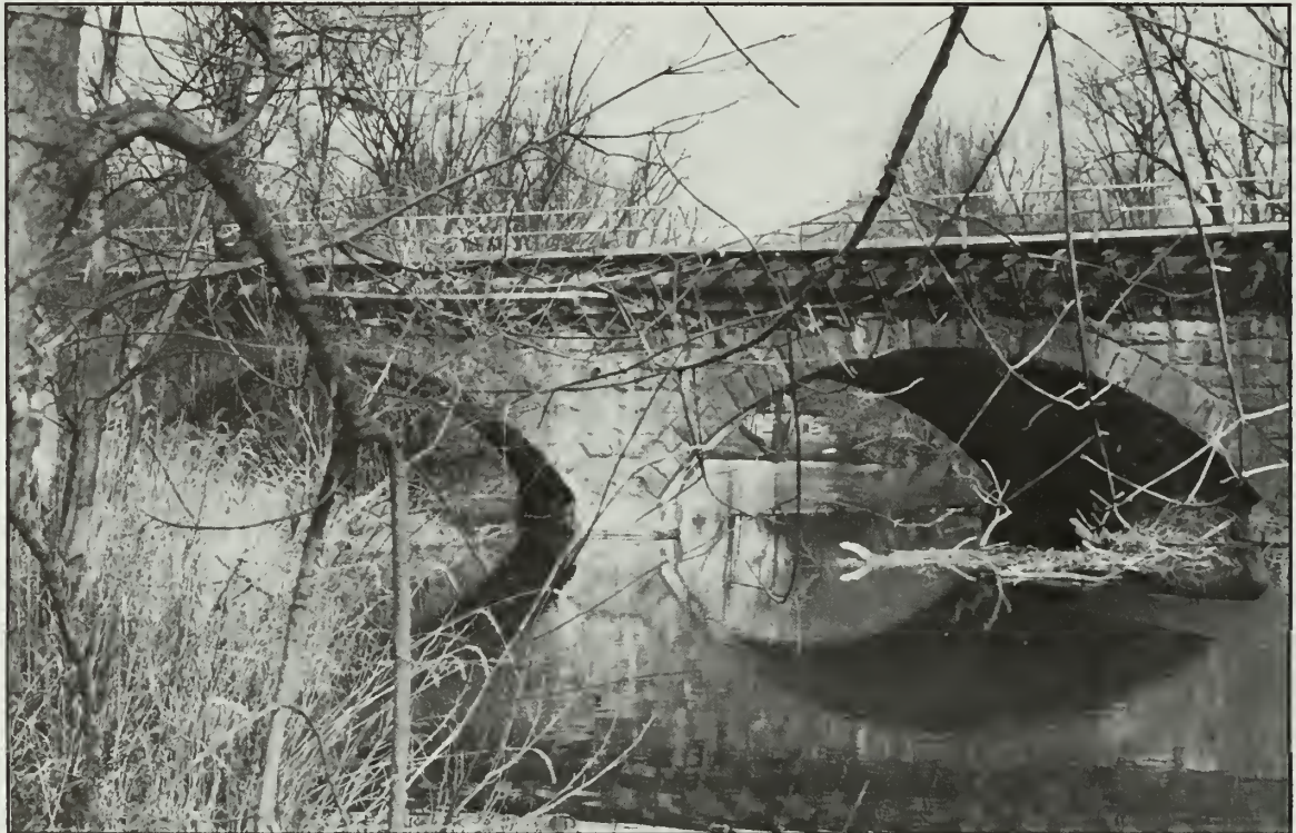
Photo 36. Pennsylvania Railroad Bridge over Shaver's Creek.
