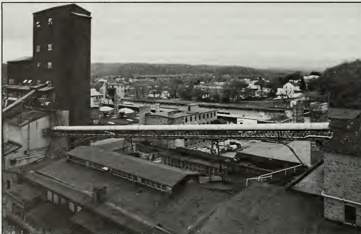
Photo 3. Harbison-Walker Refractories plant. Photo by Jet Lowe.
