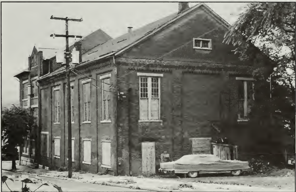
Photo 103. J. B. Kunz Company building, view along Fifth Street.
