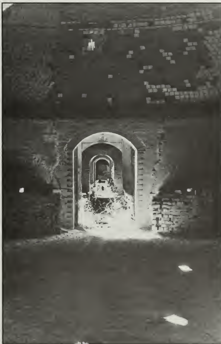
Photo 82. Interior of Harbison-Walker beehive kiln, looking through a series of kiln openings.
