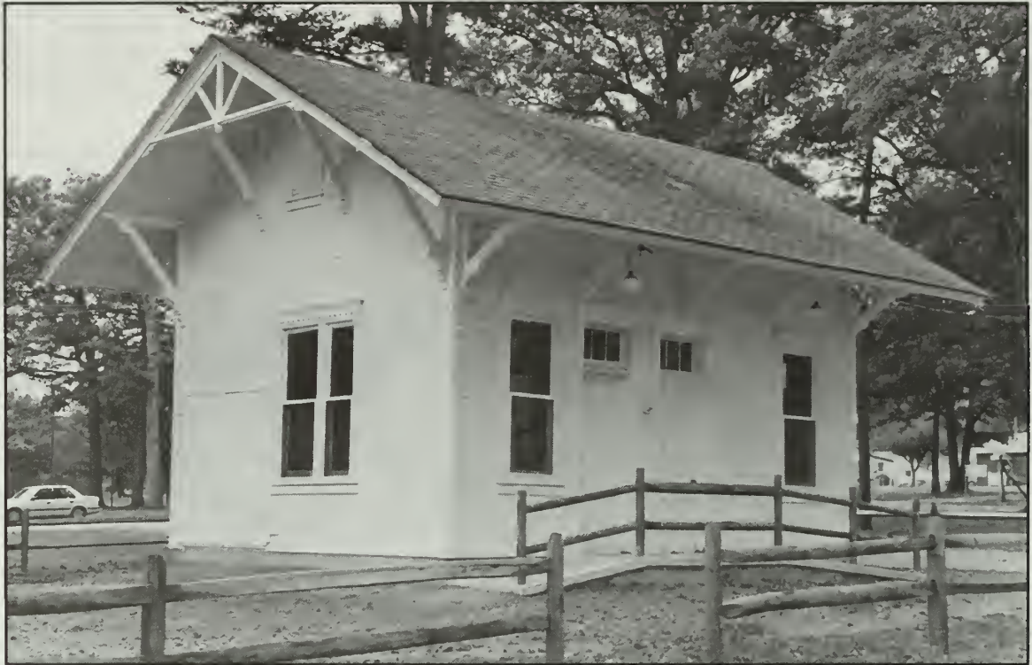
Photo 26. Long Siding Station of the Huntingdon & Broad Top Mountain Railroad.
