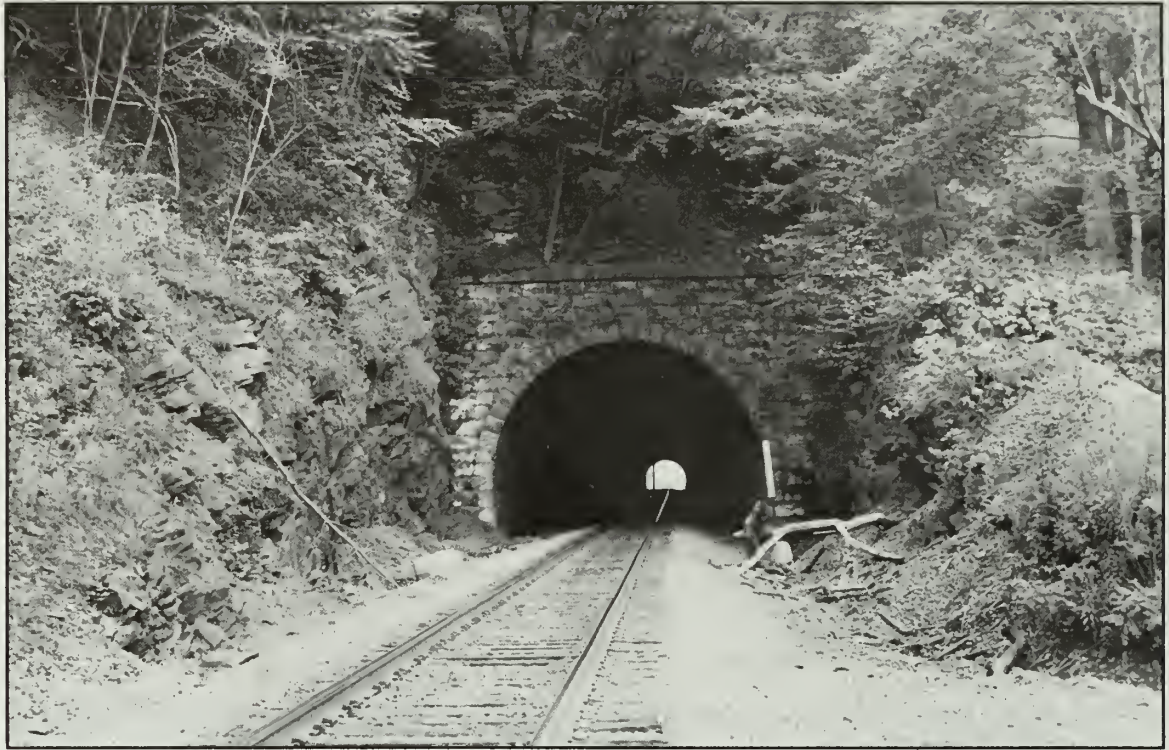
Photo 41. East portal of the PRR's Spruce Creek Tunnel.
