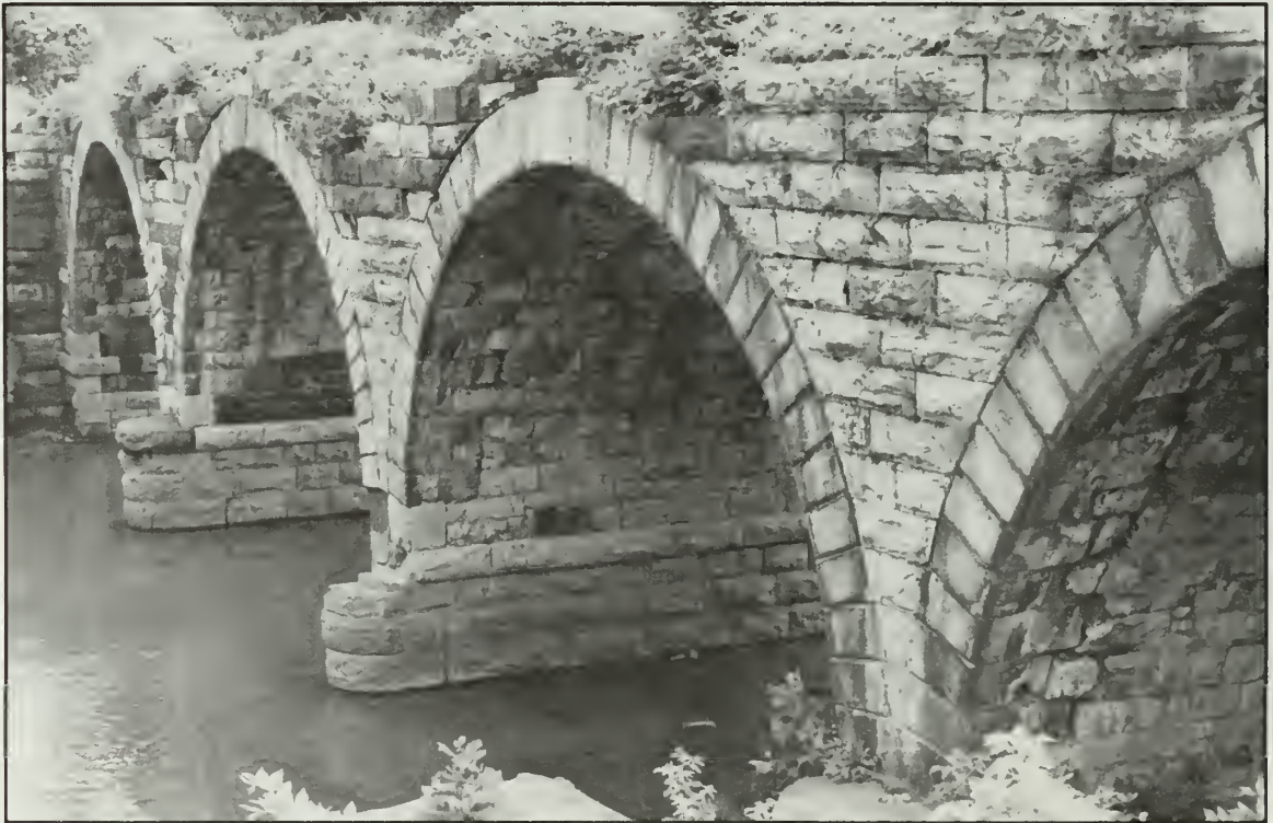
Photo 40. PRR bridge over Stone Creek.
