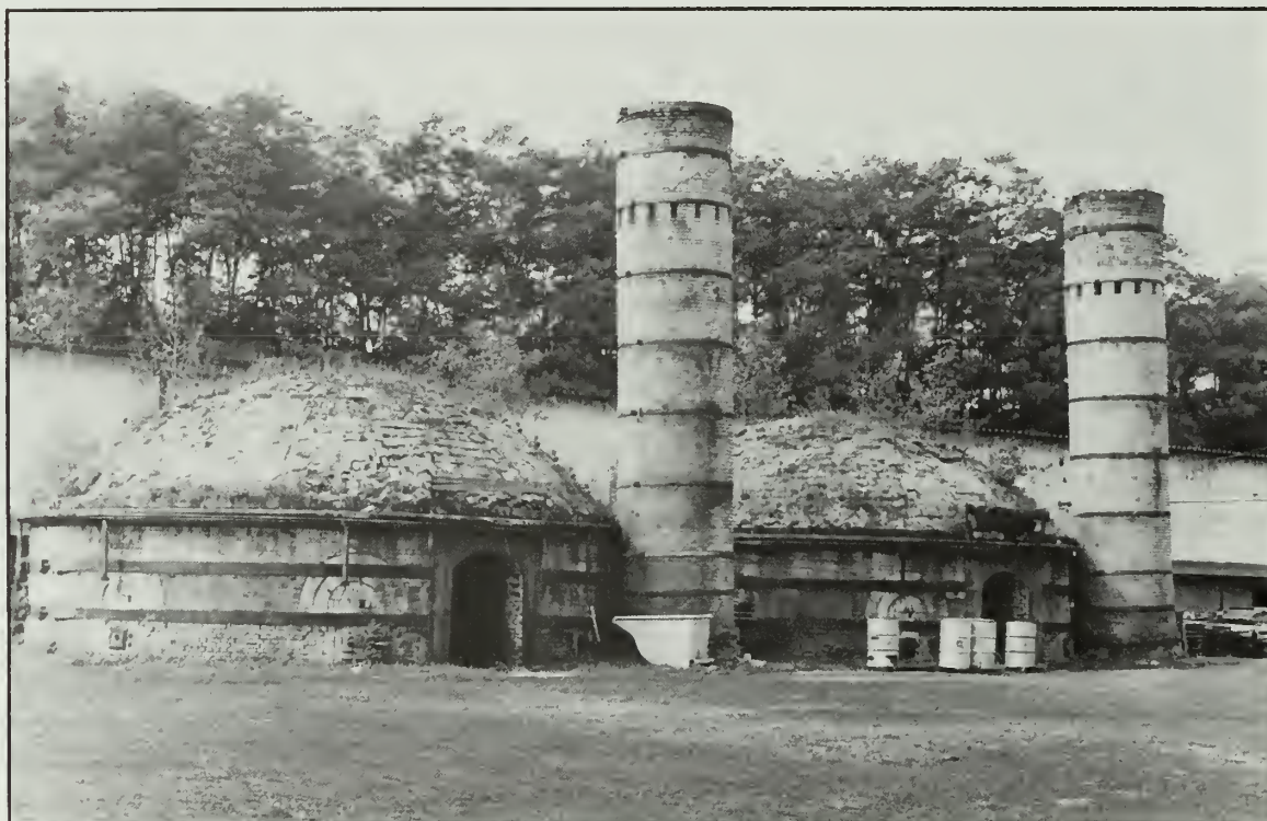
Photo 88. The two remaining beehive kilns at North American Refractories Company.
