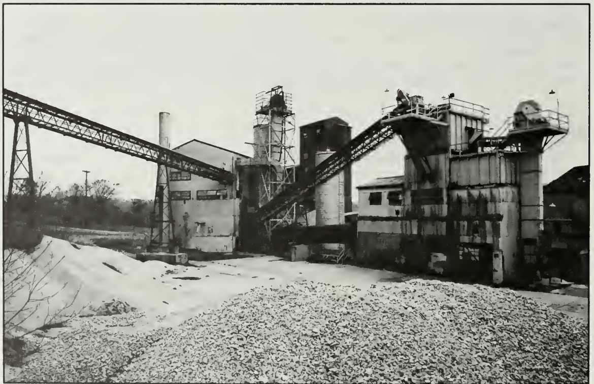
Photo 81. Harbison-Walker, rotary drier and storage silos. Photo by Jet Lowe.
