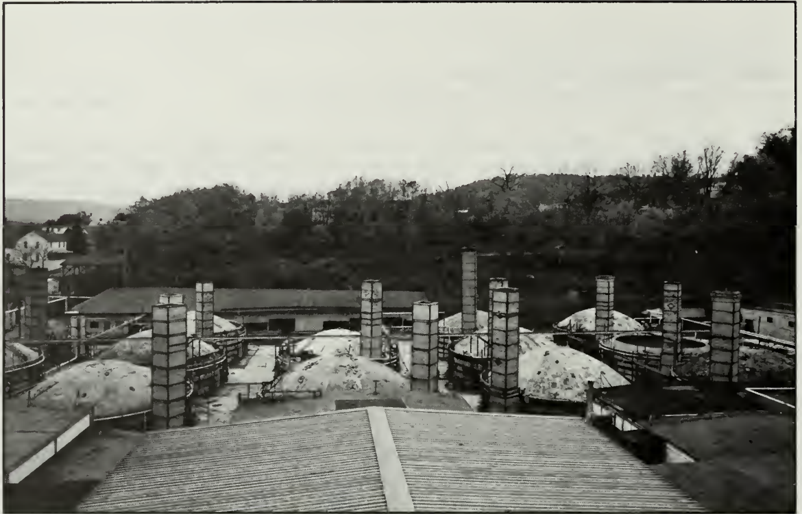
Photo 80. Harbison-Walker No. 2 kilns from the dry grind building. Photo by Jet Lowe.
