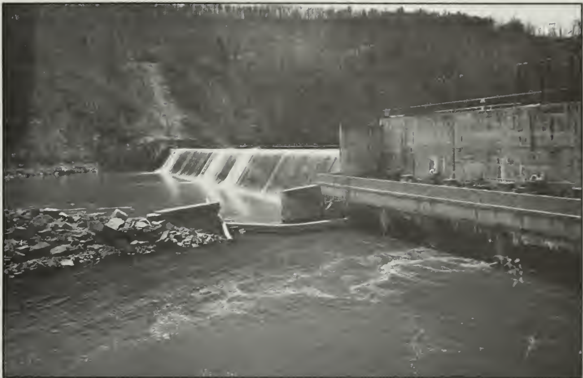
Photo 111. Warrior Ridge Power Plant, spillway and Ambursen dam. Photo by Jet Lowe.
