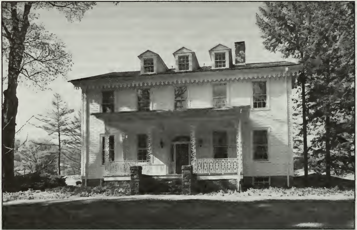
Photo 15. Ironmaster's mansion, Huntingdon Furnace. Photo by Jet Lowe.
