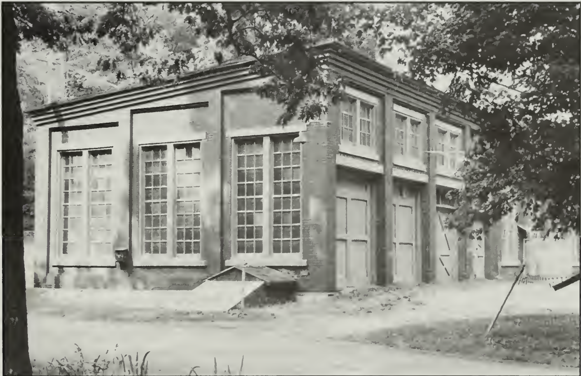
Photo 107. Bald Eagle Water Company, Pumping and Chlorination Station.
