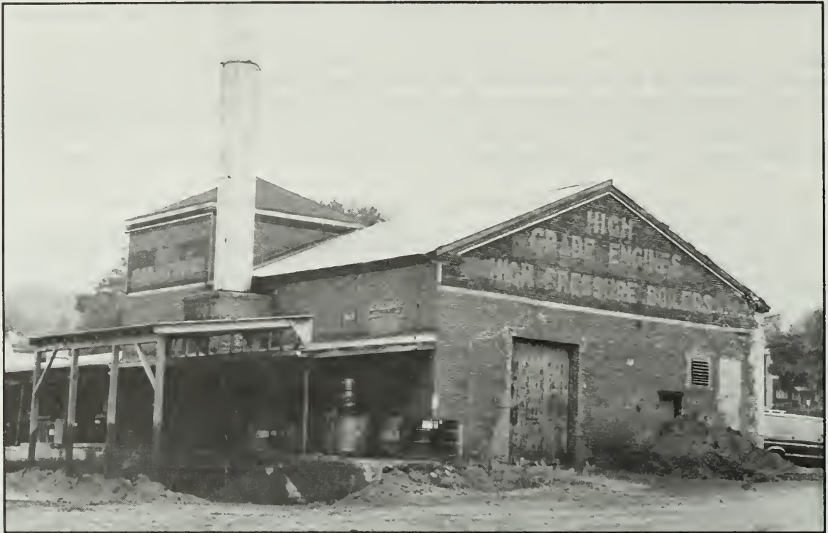
Photo 102. Huntingdon Car and Wheel Works, rear view of Powerhouse.
