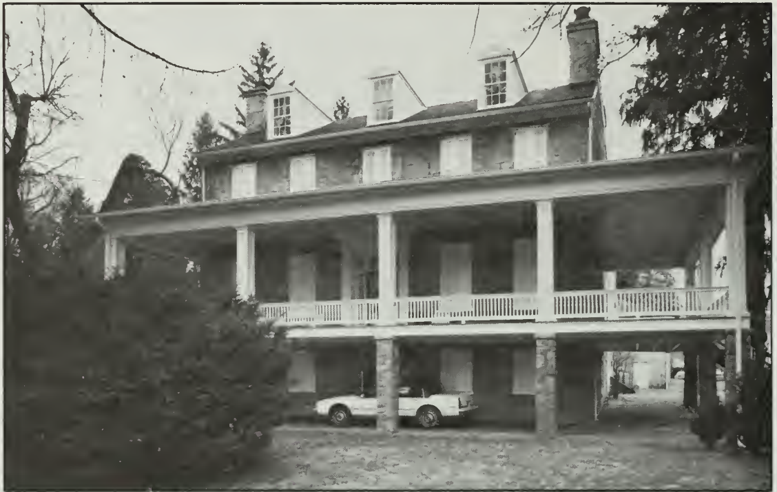
Photo 20. Pennsylvania Furnace, ironmaster's mansion. Photo by Jet Lowe.
