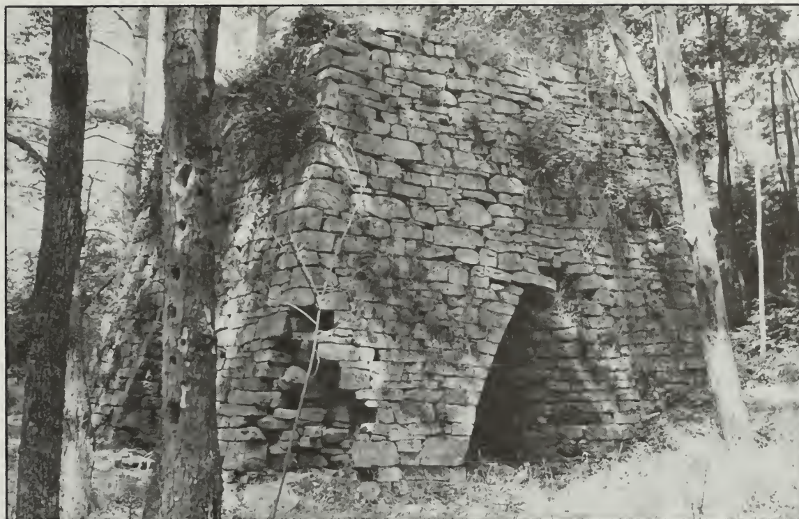
Photo 18. Monroe Furnace, view of tuyere arch.
