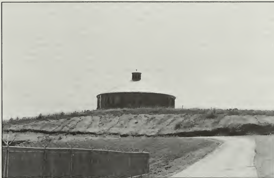
Photo 109. State Reformatory, Reservoir.
