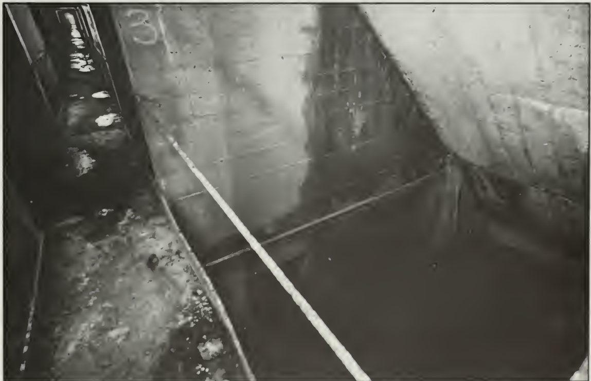
Photo 112. Interior of Warrior Ridge Ambursen dam, showing the hollow-core construction. Photo by Jet Lowe.
