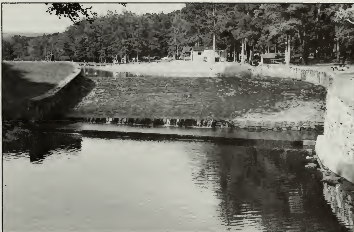
Photo 113. Whipple Dam, spillway.
