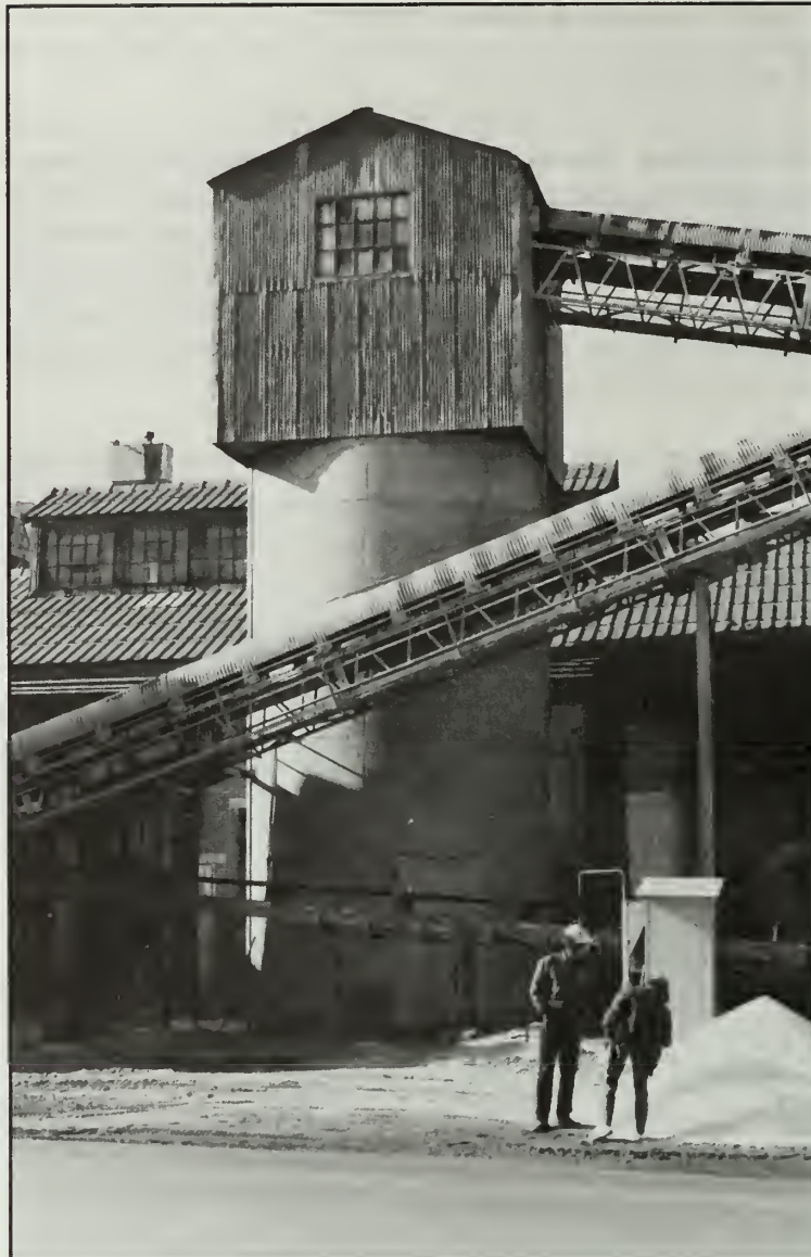
Photo 72. Storage silo at the Keystone Works.
