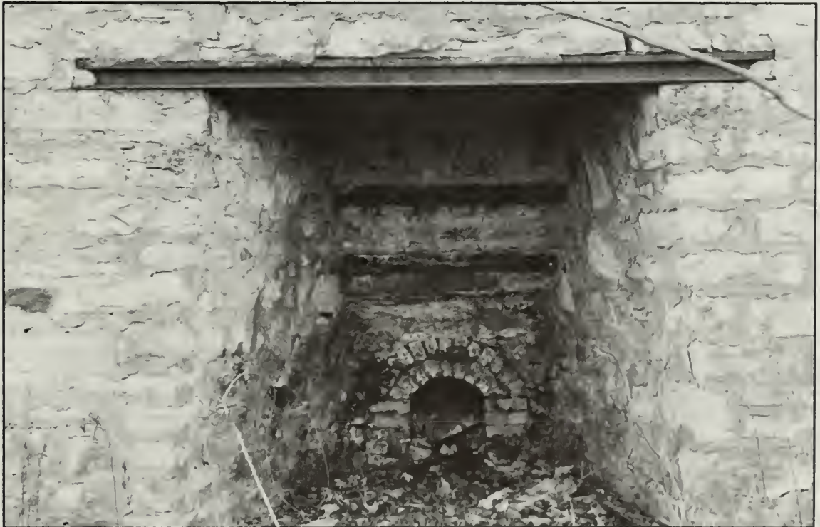
Photo 85. Detail of right opening of double limekiln.
