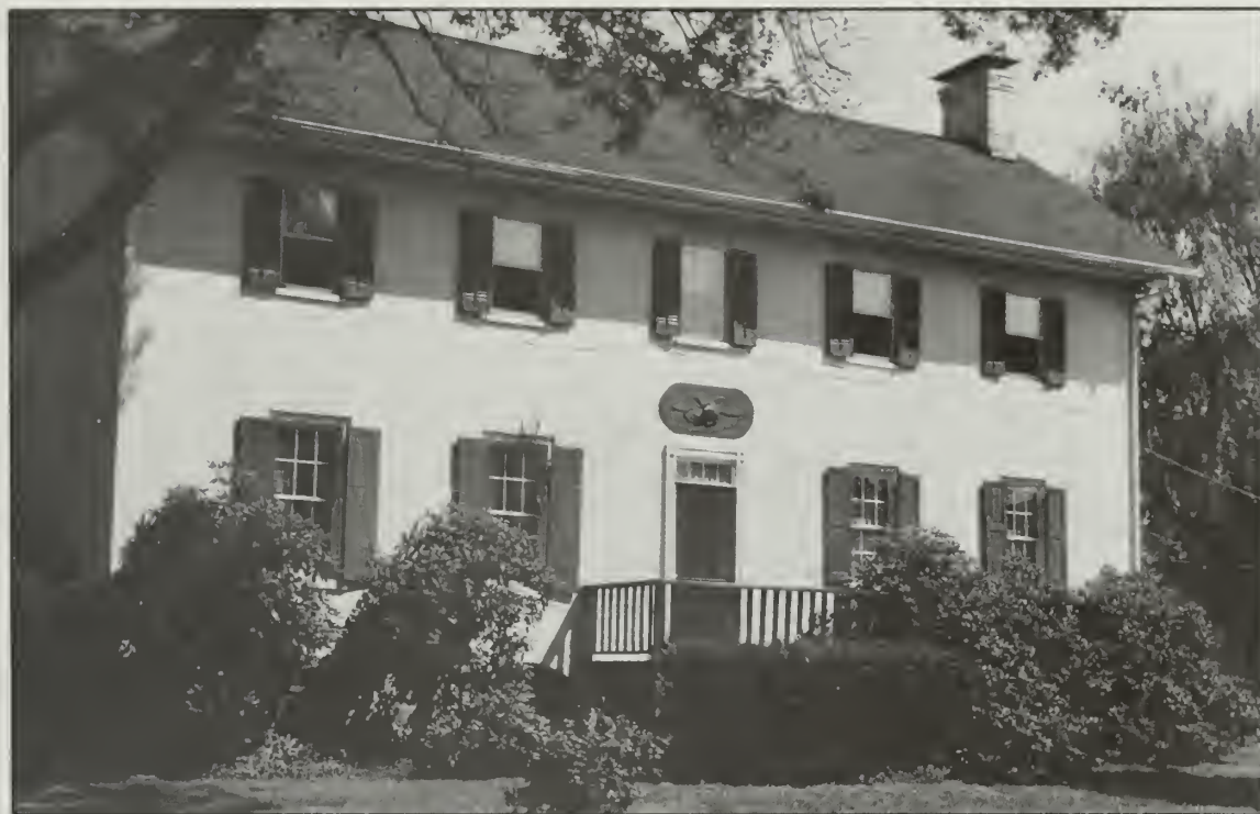
Photo 17. First ironmaster's house (1841) at Juniata Iron Works.
