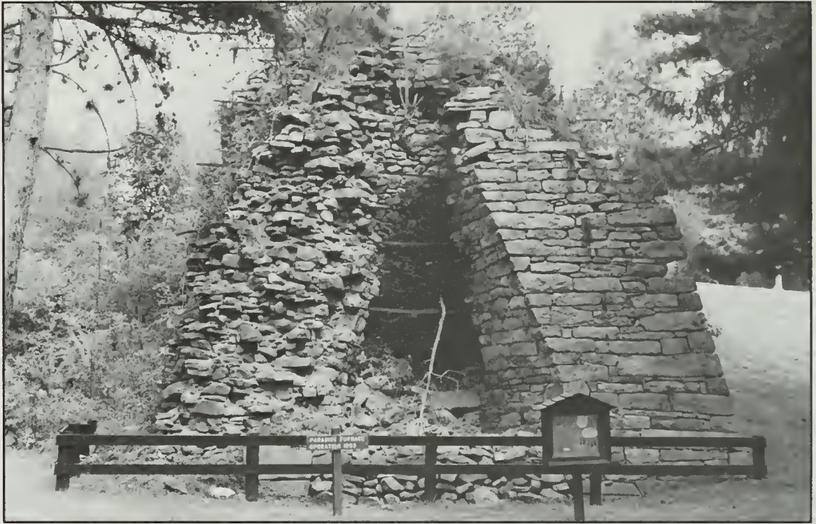
Photo 19. Paradise Furnace, view of work arch. Note support rods spanning space back of the work arch.
