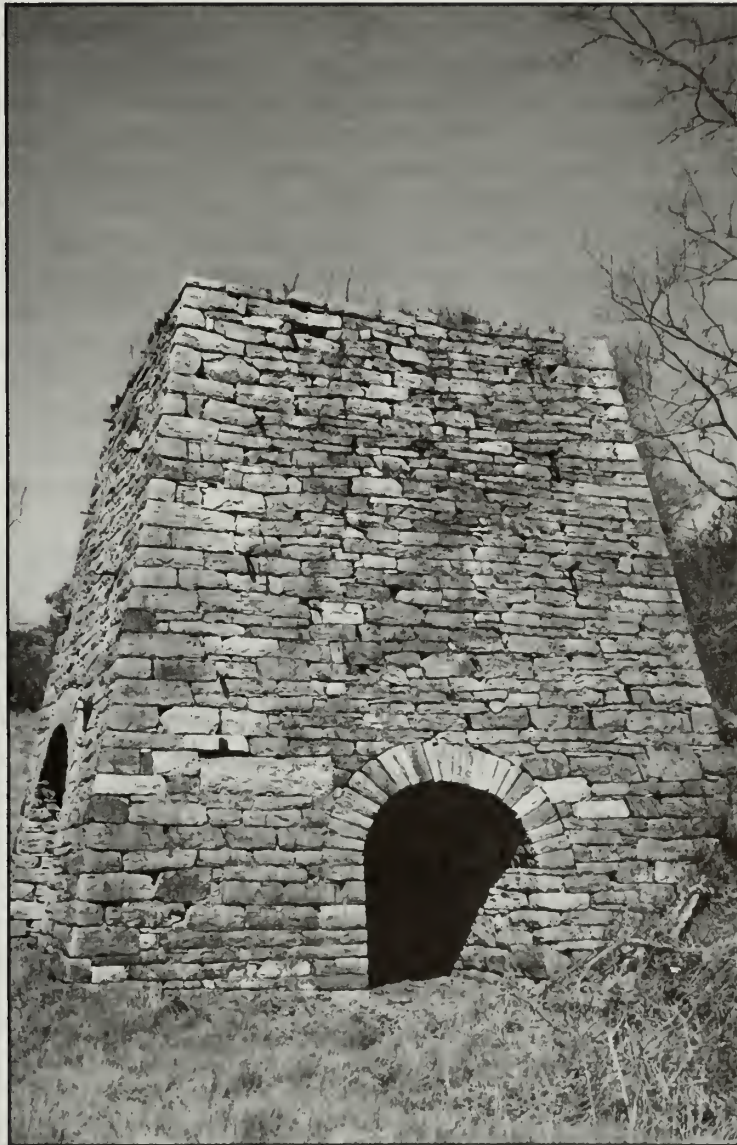
Photo 12. Huntingdon Furnace stack. Photo by Jet Lowe.
