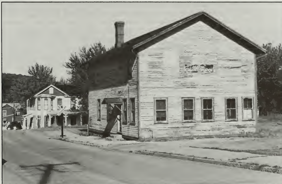
Photo 39. Mount Union Freight Depot.
