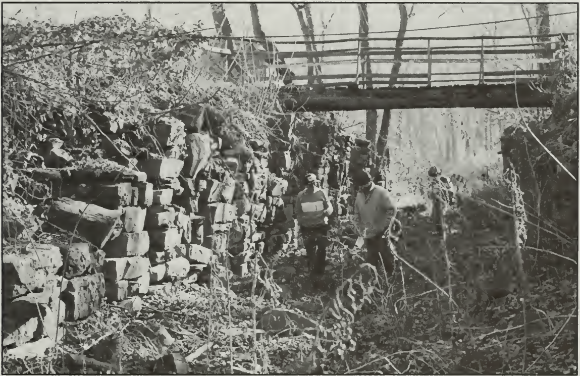
Photo 35. Pennsylvania Canal guard lock; view of east wall, looking southeast.
