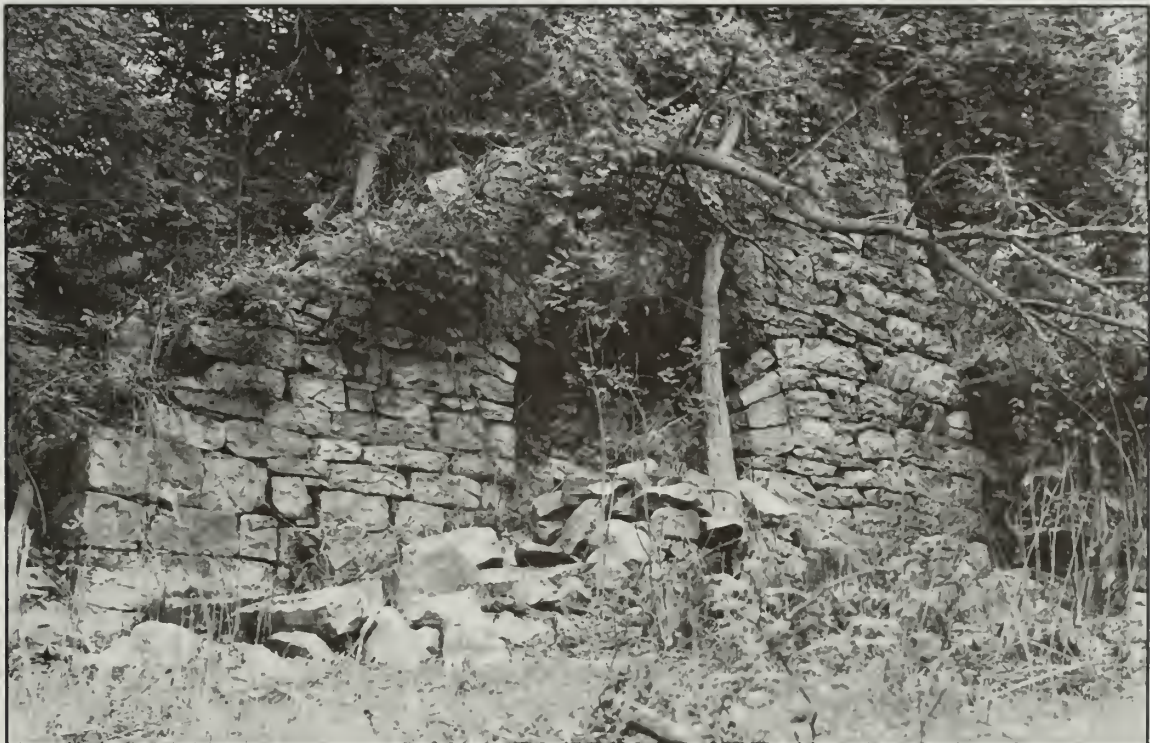
Photo 4. Remains of Barree Furnace stack, view of work arch.
