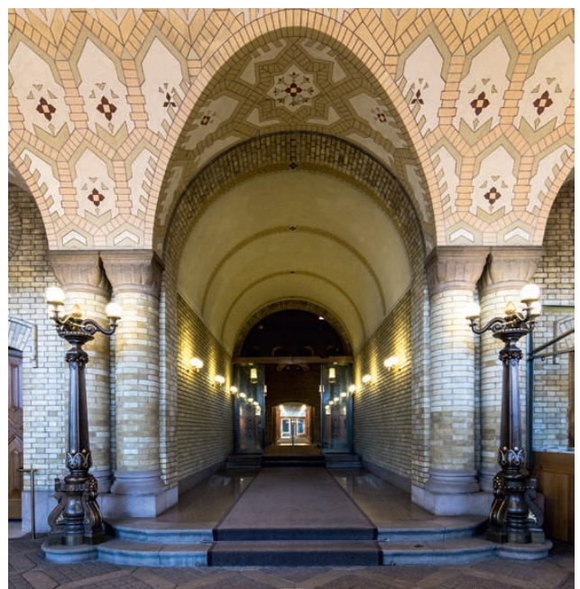
Only two steps remained of the old main staircase after the alterations. (Photo: Hans Kristian Thorbjørnsen)
