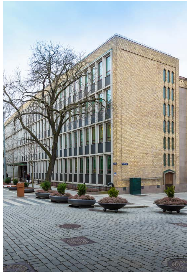
The extension facing out across Akersgata, which was completed in 1959, has a façade of light granite, highly-polished black labradorite stone and yellow brick. (Photo: Hans Kristian Thorbjørnsen)
