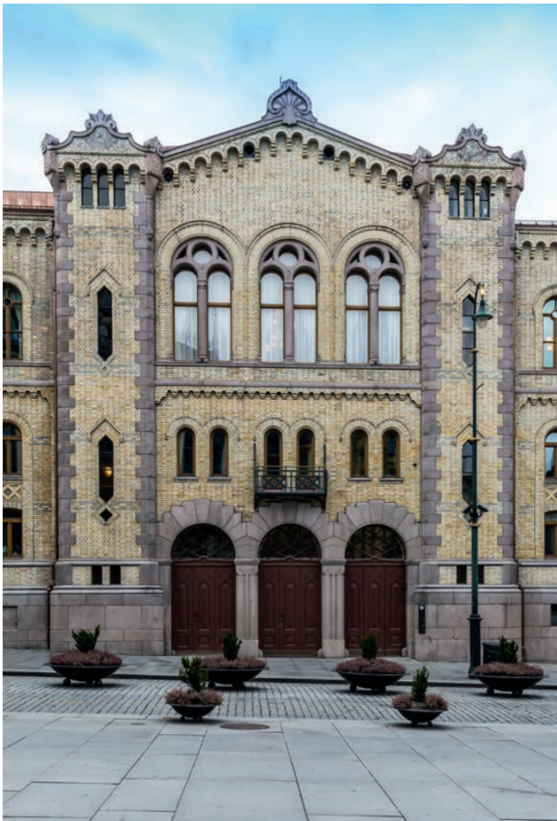
The protruding centre part of the façade facing out across Karl Johans gate marks the end of the cross-wings. The three doors are the public entrance to the Storting Chamber. (Photo: Hans Kristian Thorbjørnsen)
