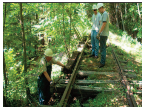
CMRR volunteers stabilize the track above Butternut Cover so that our light maintenance equipment can operate through this area to help with restoration and repair of this significant drainage culvert along the railroad.
