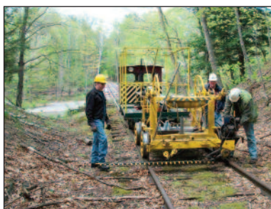
The sickle bar cutting crew ran from Shokan to the Boiceville Bridge (C30) on May 7, cutting vegetation that we had missed last year. Pictured are Bill Brosnan, George Cook and Paul Sternitzke. The crew has just turned the machine and is readying it for its return to Shokan to cut vegetation along the south rail.
