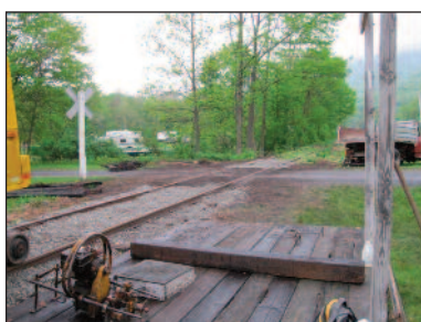
On May 14, volunteers rebuilt the private crossing at Sleepy Hollow Campground.
