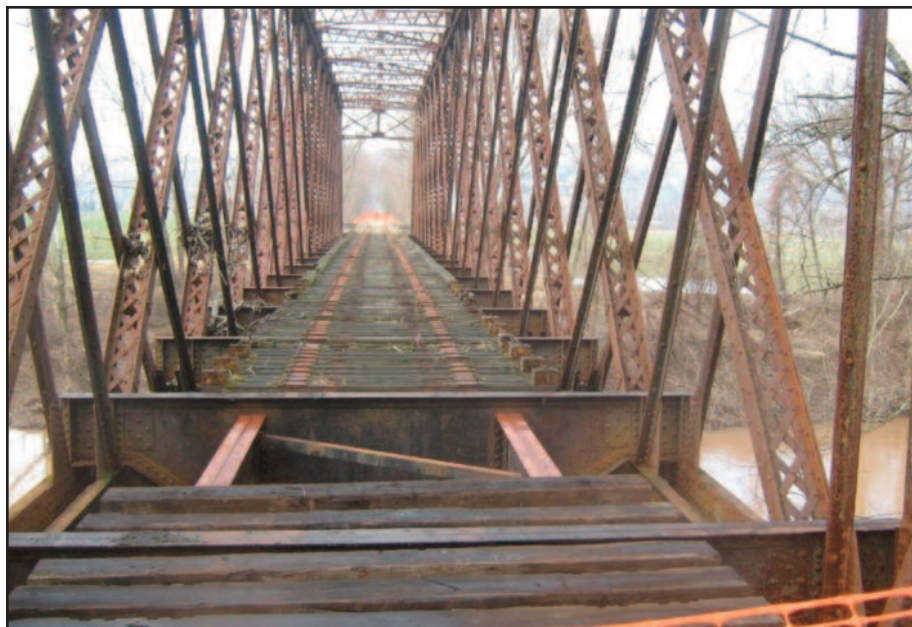
Bridhe C9 in Kingston with the first new timbers in place.
