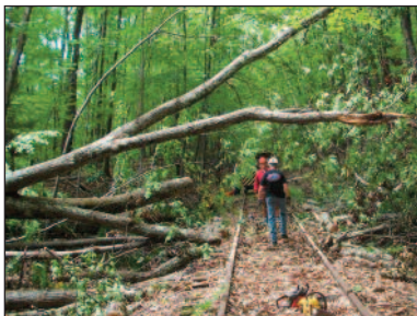
The brush crew removed trees downed by Hurricane Irene seen here at MP 14.4. This was typical of the damage we encountered in this section of the line on September 17.
