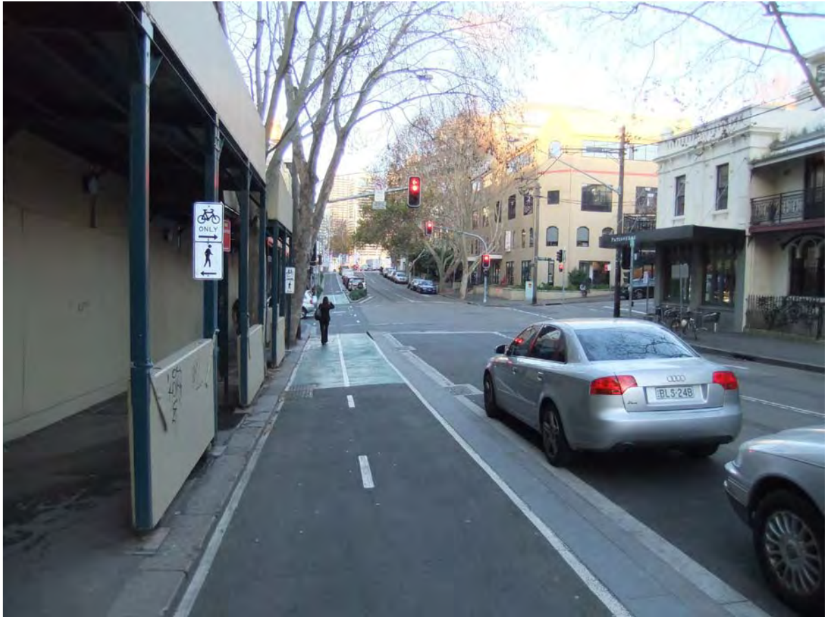
Figure 3.11 Union Street looking east
