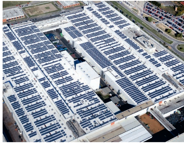
Late in 2013, SEAT brought the auto industry's largest roof-mounted photovoltaic plant "SEAT al Sol" on stream in Martorell (Spain).
