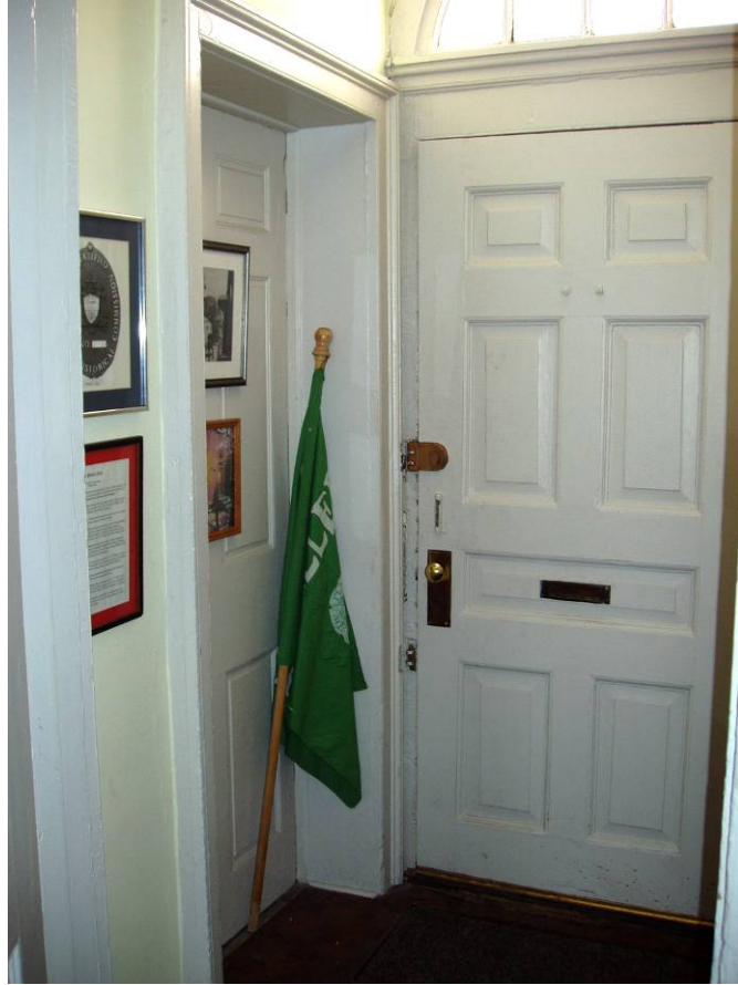
Figure B76. First floor entrance vestibule, looking southwest. Note the door between the two houses inserted at the left, but seemingly never used.
