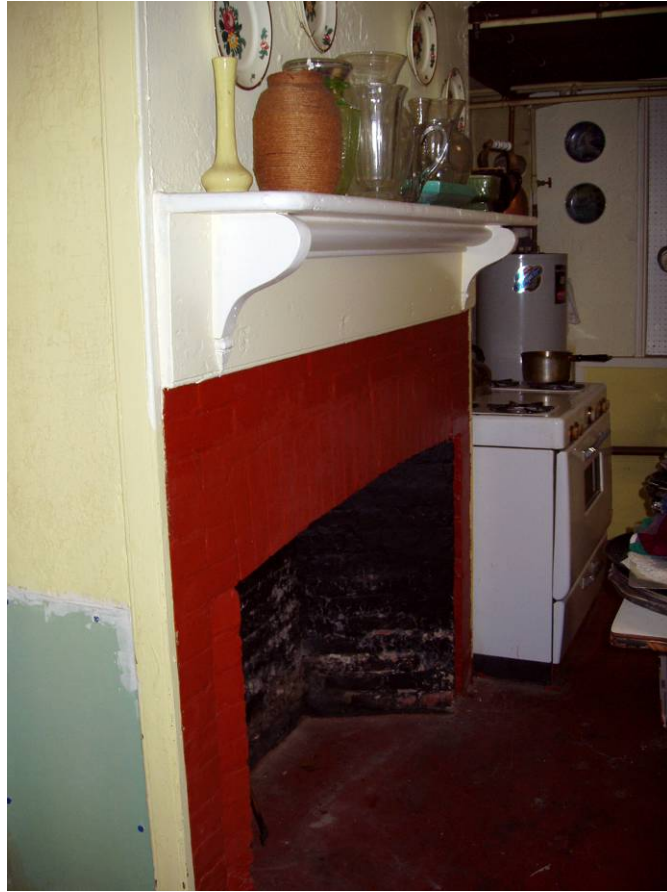
Figure B42. Basement, kitchen fireplace. Note the sheetrock patch at the lower left on the wall.
