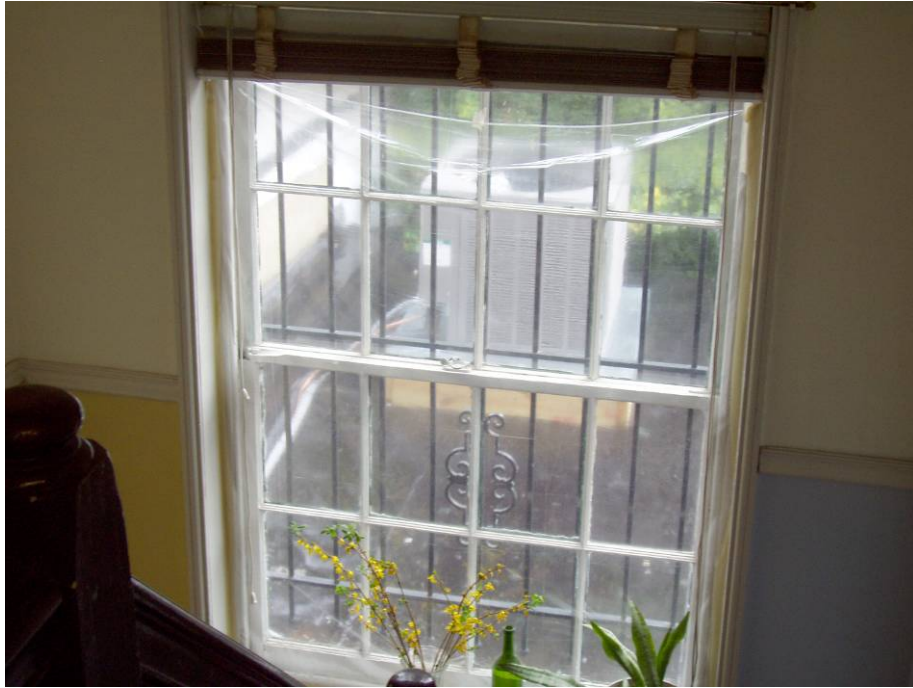
Figure B81. Window at stairway landing. Note the HVAC chiller on the roof of the first floor restroom just outside the window.
