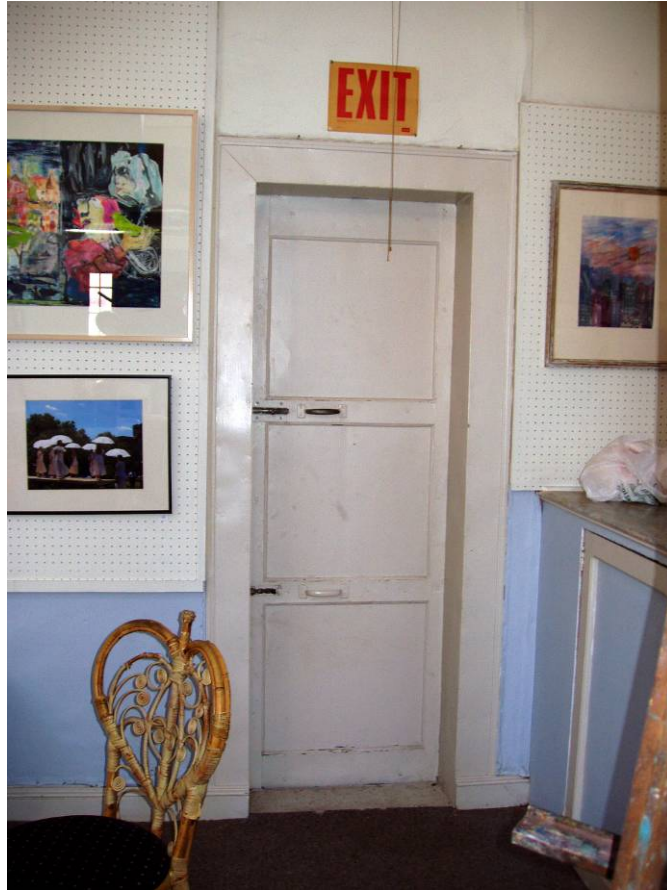
Figure B84. Second floor studio exit door, southeast corner.
