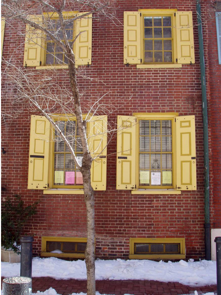
Figure B7. Exterior façade of 247 S. Camac Street, southern half (former 249 S. Camac Street). Note slight discoloration in the mortar on the right side, where the front door of 249 S. Camac Street was removed.
