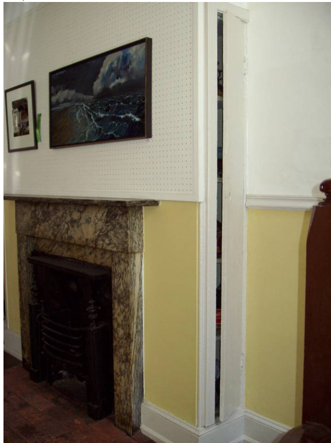
Figure B54. First floor main room, northeast fireplace. Note the original cabinet along the side of the fireplace extension.
