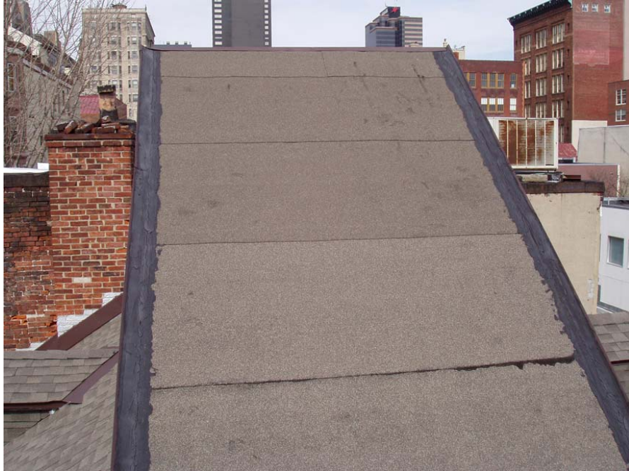
Figure B103. Back of the skylight, looking north.
