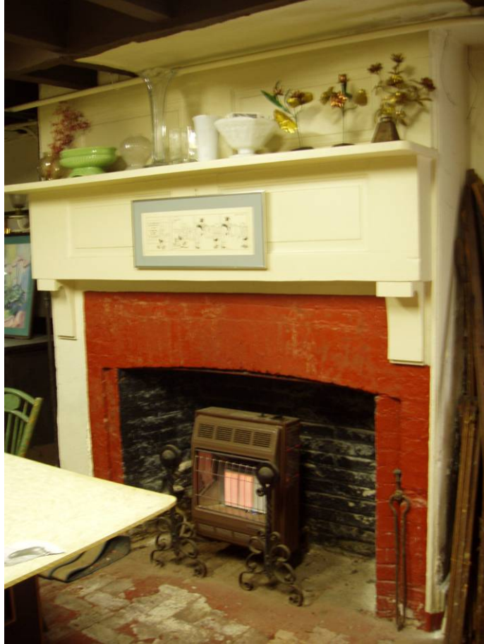
Figure B33. Basement main room, fireplace. Note the gas-burning space heater installed in the fireplace.
