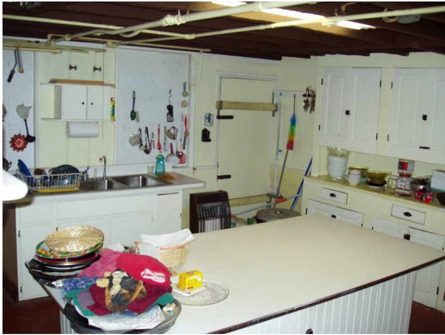
Figure B43. Basement kitchen, looking southeast. Note the pegboard covering the original windows behind the sink.
