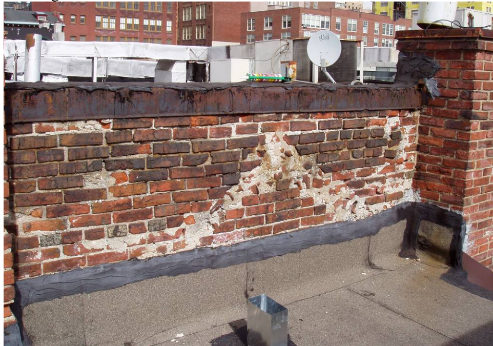
Figure B100. Roof and north party wall. Note the outline of the original roof of the building and the opening in the roof for the HVAC pipes.
