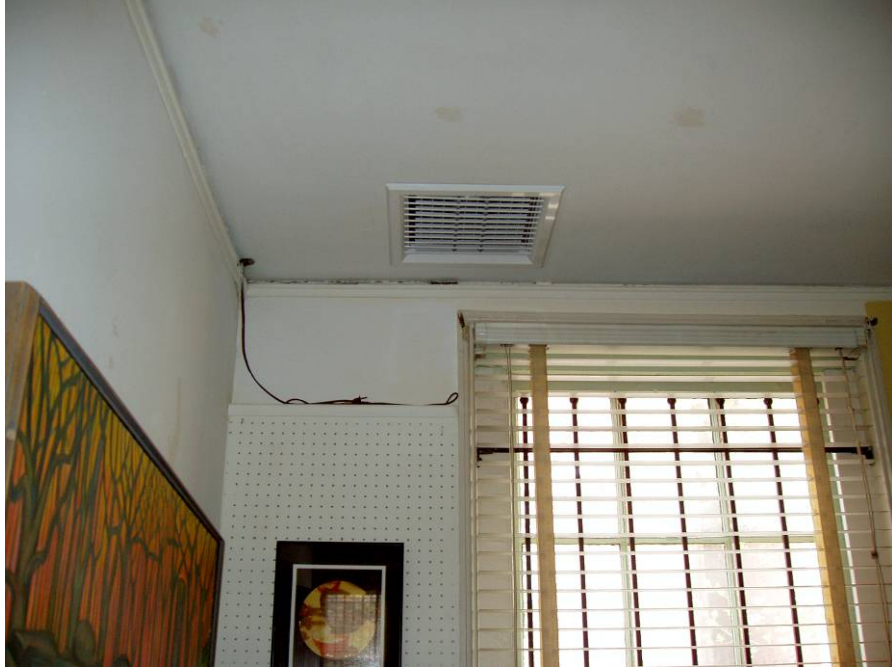
Figure B55. First floor main room, northwest window and vent in the ceiling.
