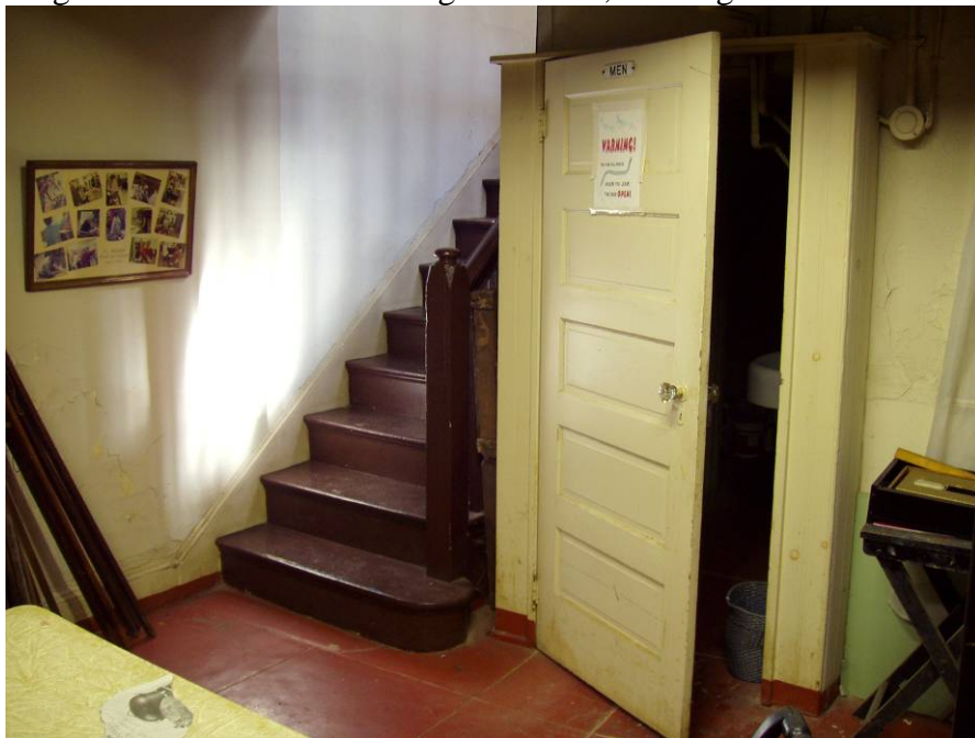
Figure B27. Basement main room, looking northeast to the stairs and the restroom. Note the green panel of sheetrock patching at the lower portion of the wall to the right.
