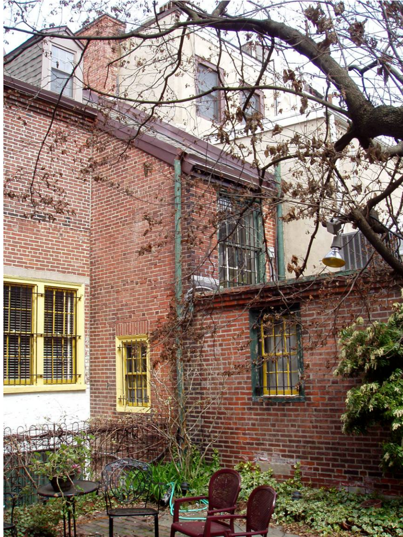
Figure B14. Rear façade, north end, showing the rear stairwell and restroom extension.
