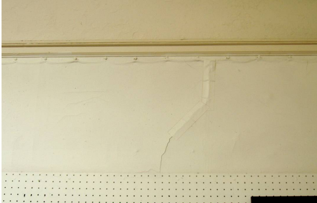
Figure B93. Second floor studio, upper portion of the south wall at the west, showing the early monks' cloth under layers of paint.
