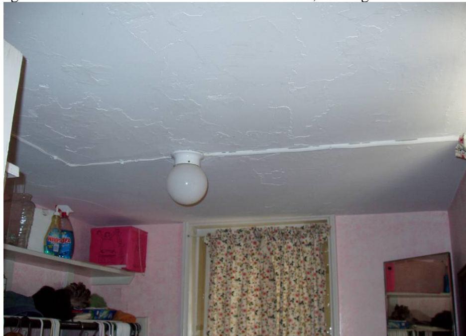
Figure B59. First floor restroom in rear extension, ceiling and electrical wiring.
