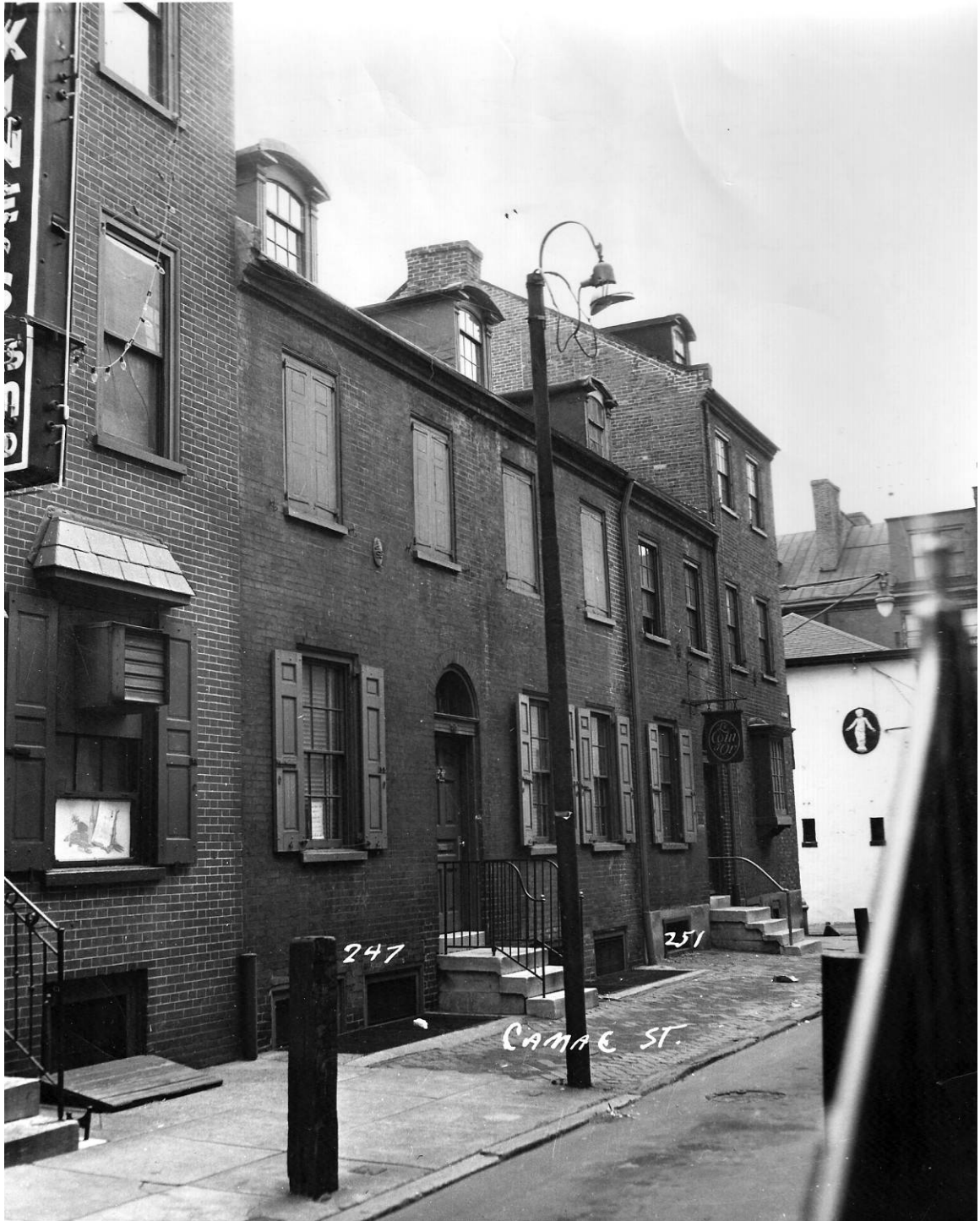
Figure A23. Photograph of the Plastic Club, 1959. Note the dark color of the exterior woodwork, the sunken lightwells at the basement level, and the closed shutters at the second floor. (Source: Plastic Club Archives)
