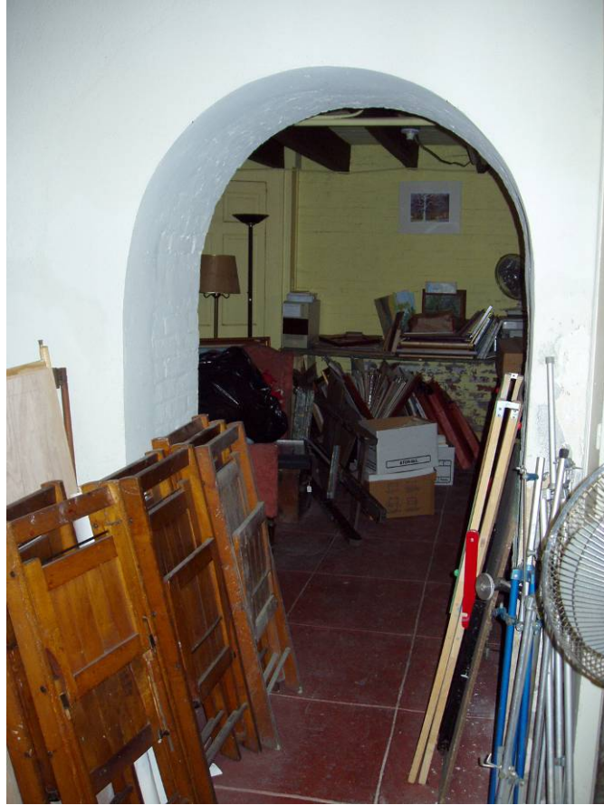
Figure B36. Basement main room, looking south into the office.
