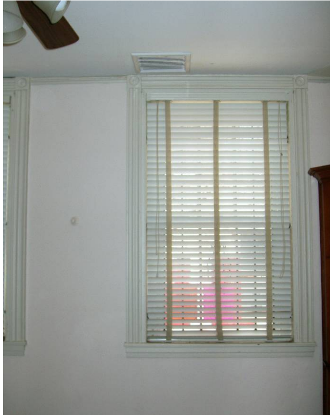
Figure B69. First floor Board Room, northwest window with vent in the ceiling.
