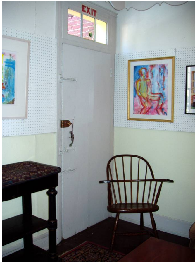
Figure B73. First floor tea room, southeast corner. Note metal security door and bulls-eye glass in transom above.
