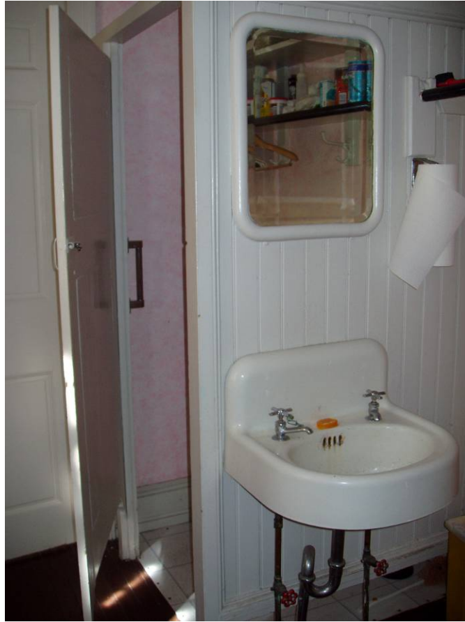
Figure B62. First floor restroom, northwest corner, original sink and toilet enclosure.
