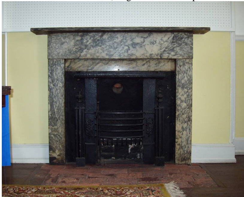
Figure B52. First floor main room, northeast corner. King of Prussia marble mantle dates to 1840s with original coal stove.
