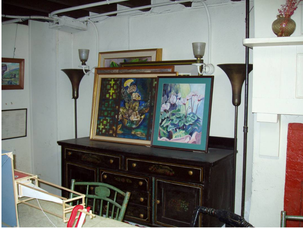
Figure B32. Basement main room, north wall. Note the original gas wall fixtures, updated for electricity.
