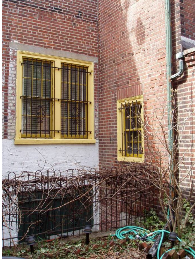
Figure B16. Rear façade, northern end and rear stairwell extension.
