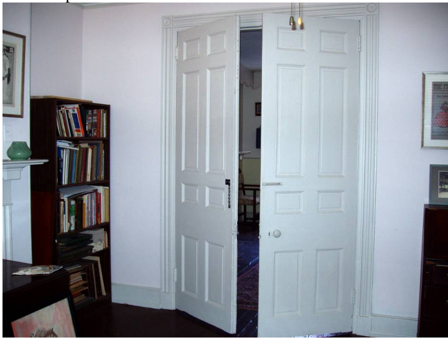
Figure B64. First floor Board Room, looking northeast.
