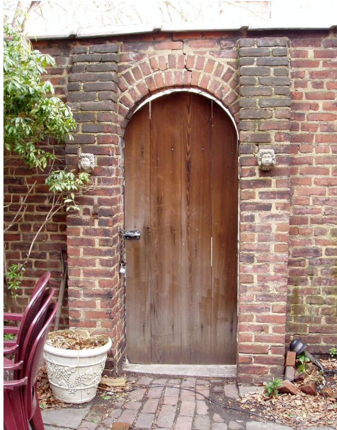
Figure B26. Rear door of the garden wall, fronting on Fawn Street.
