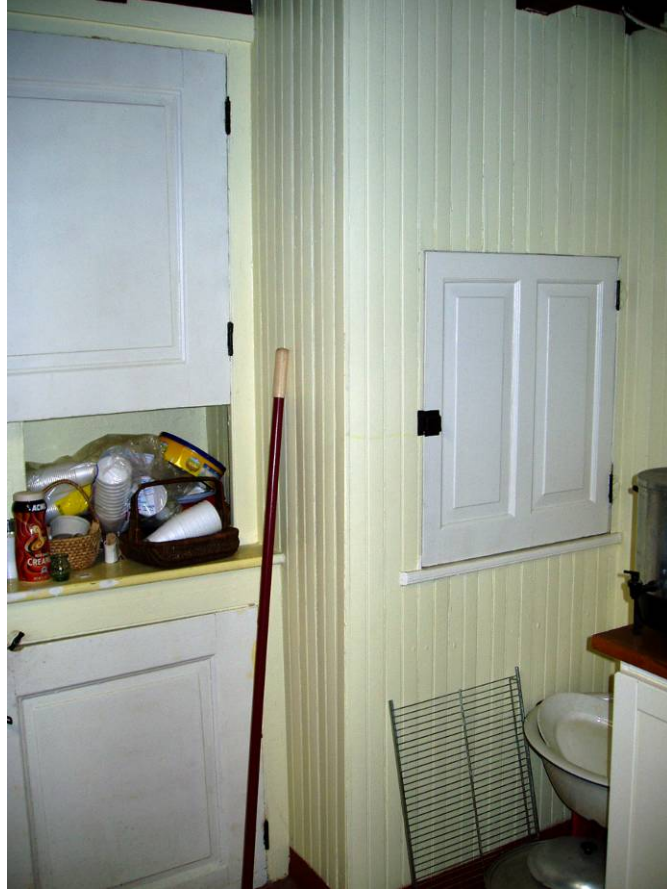
Figure B45. Basement kitchen, southwest corner, showing dumbwaiter.
