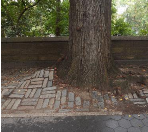
pushing up bricks
