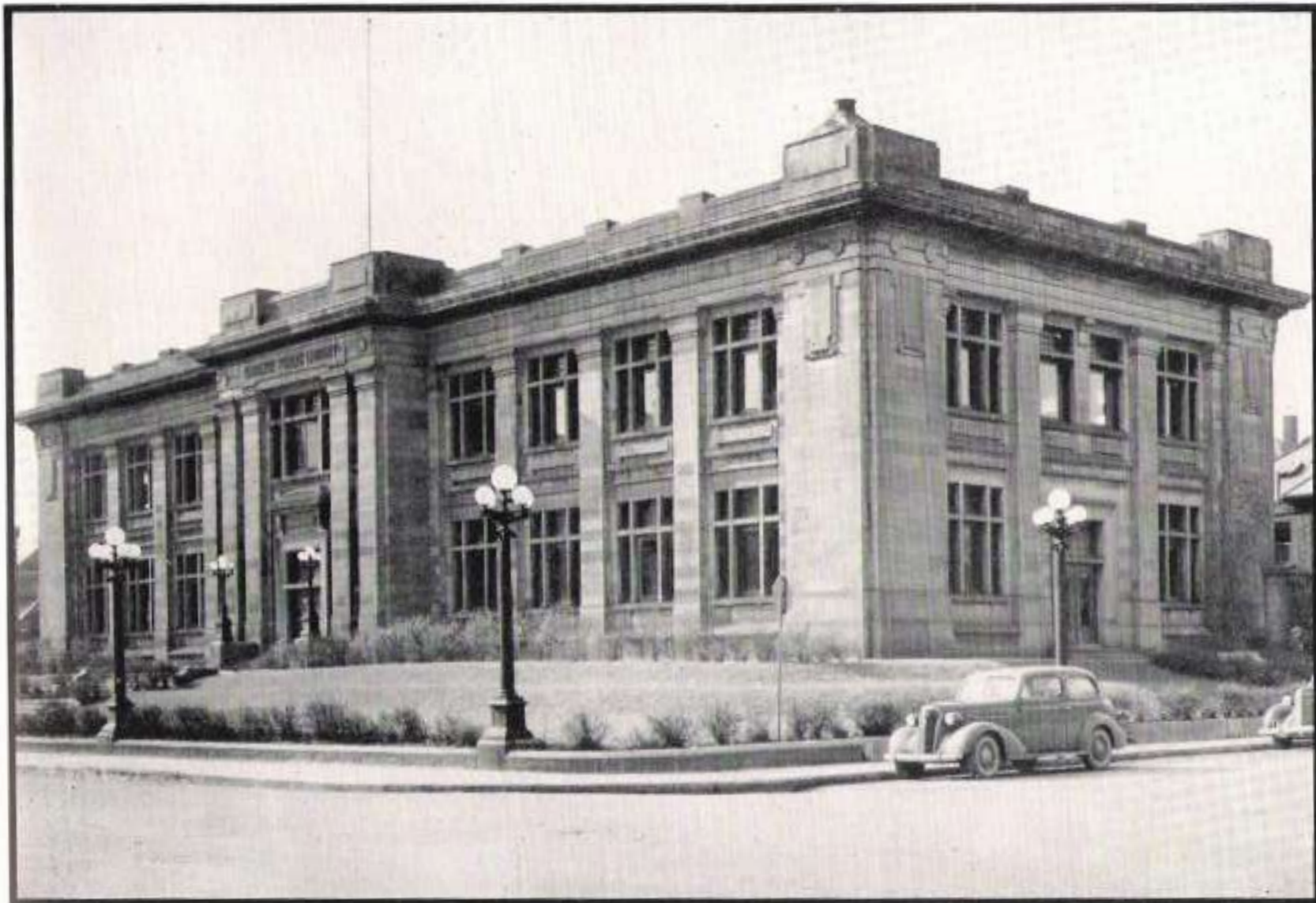
Hamilton Public (Carnegie) Library Built 1911-12. Currently – Unified Family Court. Located at corner of Main Street and MacNab Street (southwest corner).
