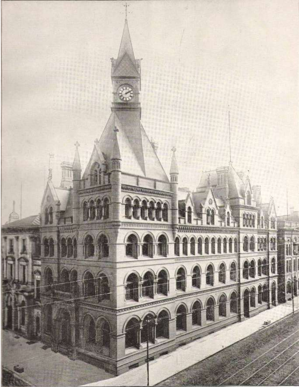
Canada Life Assurance Co. Building.
