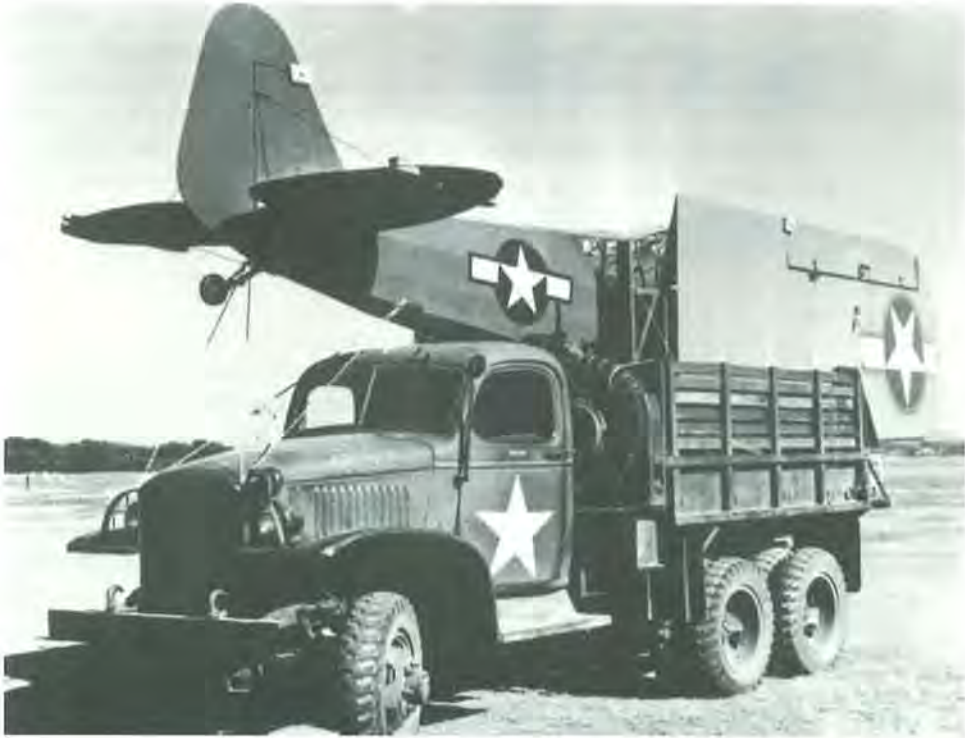
AN O-59 LOADED ON A 2½-TON 6X6 ARMY TRUCK FOR CROSS-COUNTRY MOVEMENT
