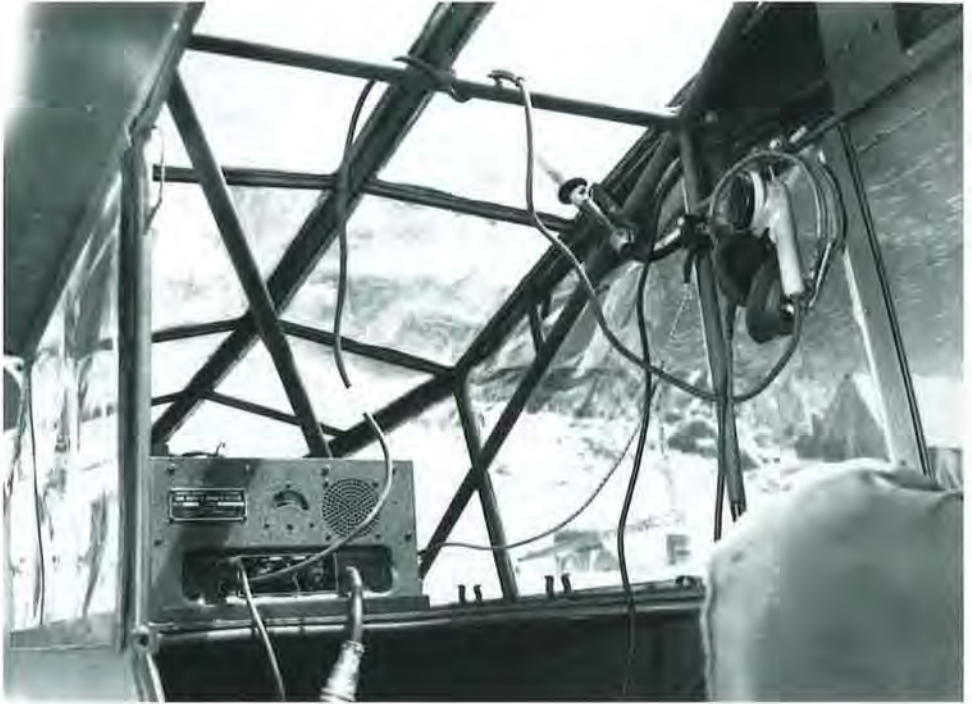
THE SCR-610, A VEHICULAR RADIO THAT SUPPLEMENTED THE SCR-609 DURING THE LATTER STAGES OF WORLD WAR II, SHOWING THE TYPICAL MOUNTING IN AN L-4
