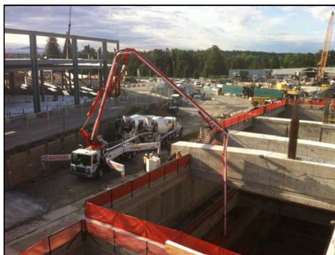
Concrete pumping at U250.
