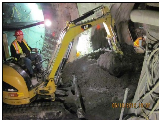
Excavator at Cross Passage #17.
