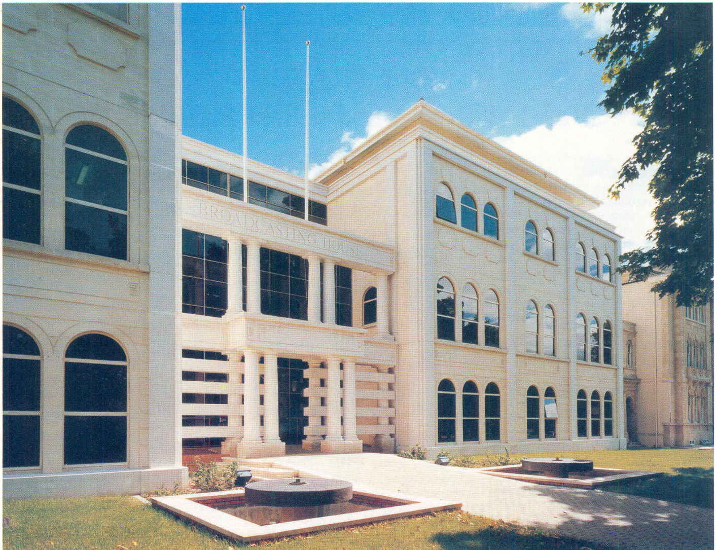
The two front villas and the entrance portico.
