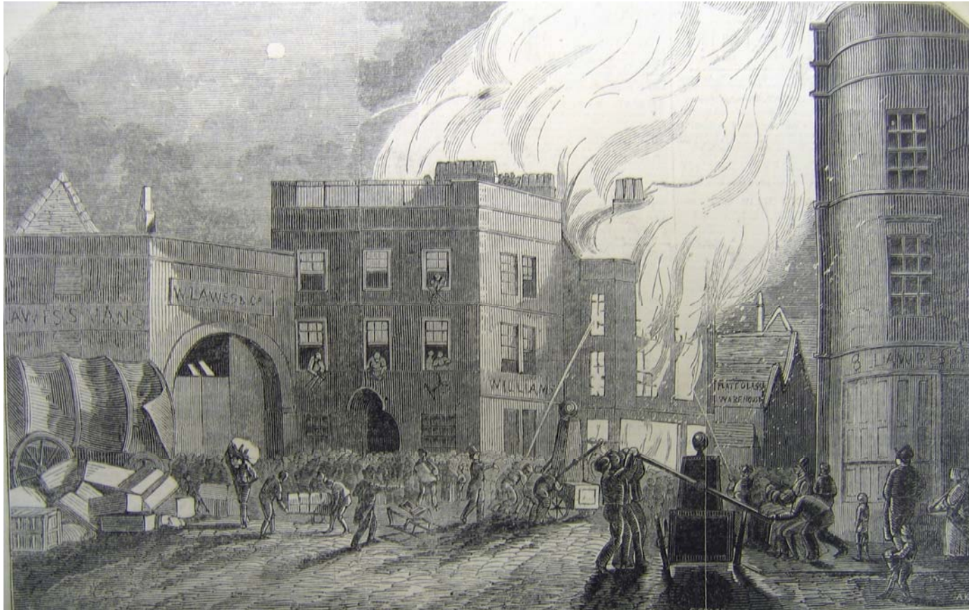
1846 Fire at The Candle Factory 4 Saw Close 258
