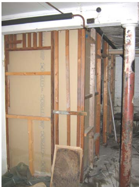
Basement 19 th century kitchen
