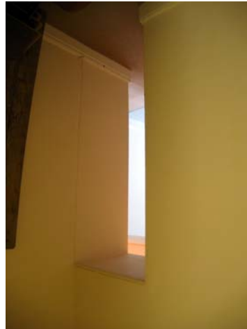
Window cut in wall [02-04]
