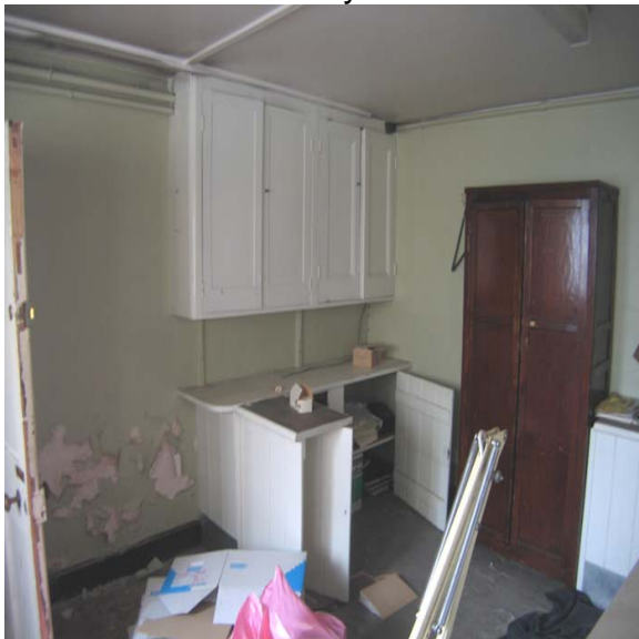
Basement 20 th century kitchen
