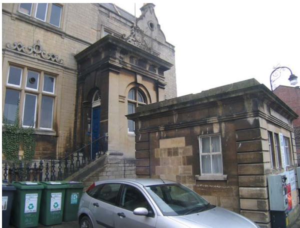
Bluecoat House from north-west and south
