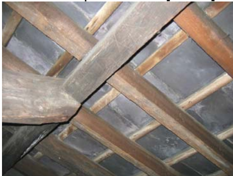
Roof space off top staircase
