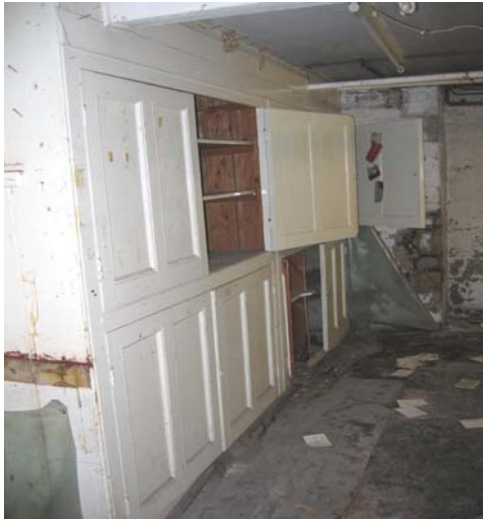
Basement 19 th century kitchen
