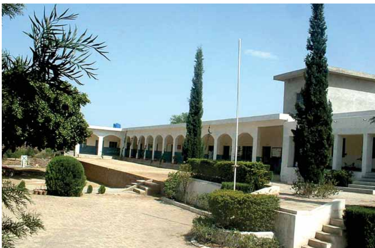
Government Boys High School Jabbar which was completely rebuilt by the Foundation was declared the Best Model School of District Rawalpindi out of 293 High schools of the District in 2009.
