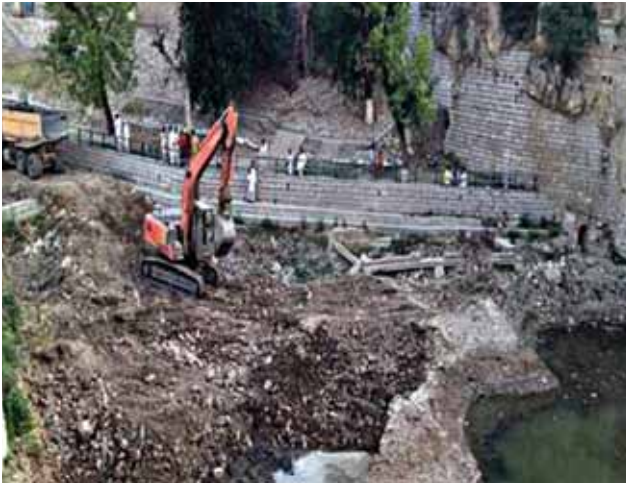
Prior to restoration
