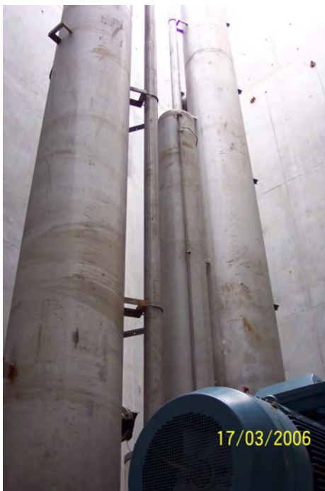
Picture 5: Biogas upgrading in Lille [LMCU].
