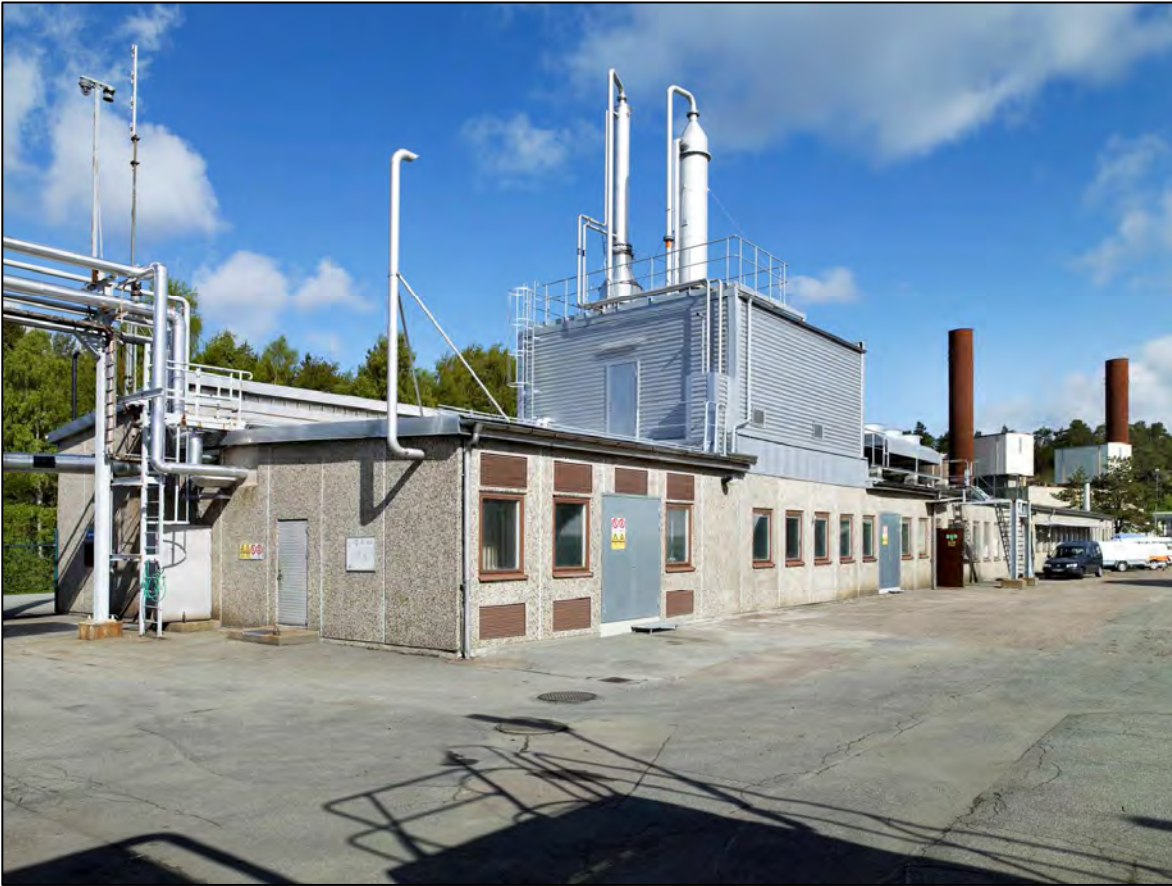
Picture 3: Biogas upgrading plant Göteborg [GE].
