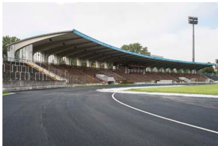
Rosenaustadion in Augsburg, Blick zur Tribüne (Foto: BLfD, Michael Forstner)
