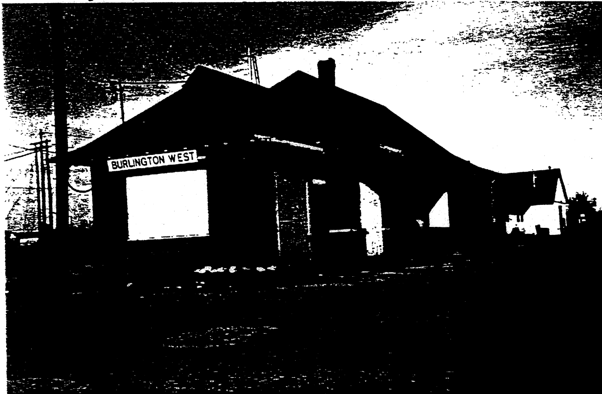
14 Burlington station, three quarter view, from the southwest, showing the characteristic profile of the hipped roof, identifiable at a distance; and the closed-in shelter at the west end. (John L. Nicholls, Analytica Associates, 1993.)
