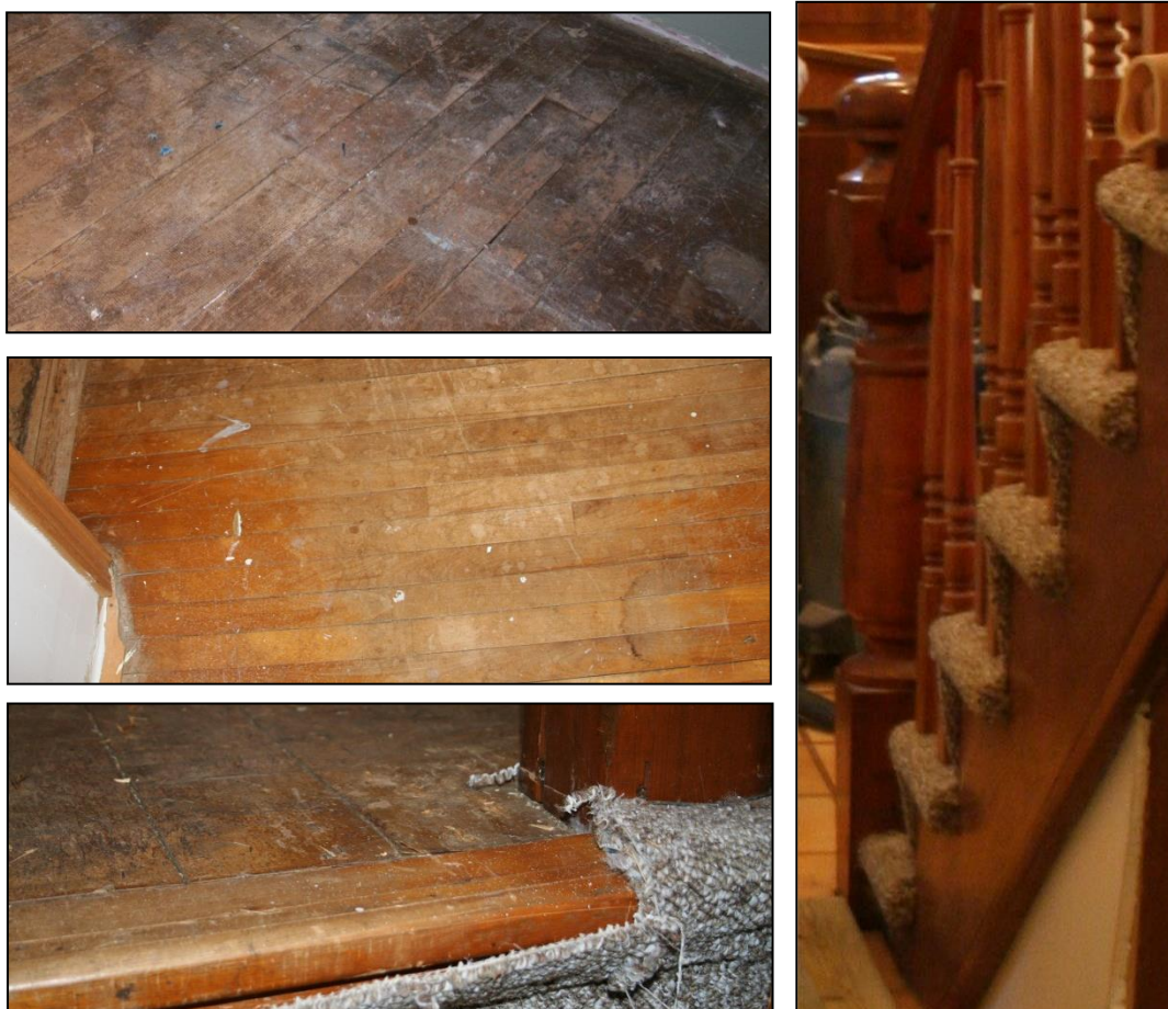
Clockwise from top left: Six-inch tongue and groove hemlock flooring in the lower storey hallway; staircase with turned spindles and butternut banister; top step of staircase; oak flooring in living room.
