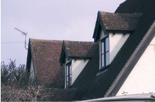
Dormer Windows - Horne Row
