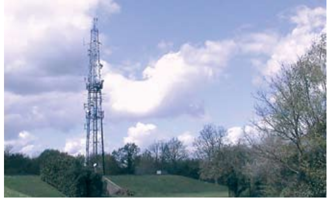
The Bakers Lane Communications Tower
