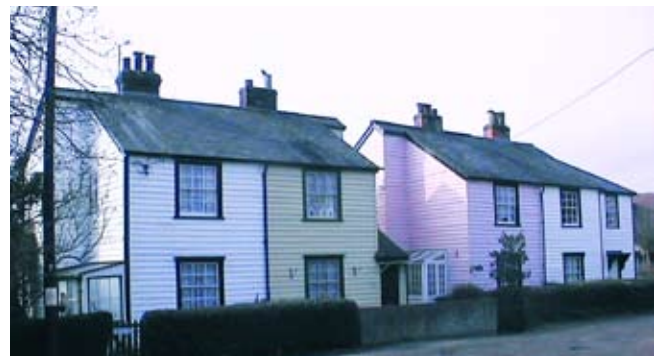
Weather boarded cottages - Plumtree Lane
