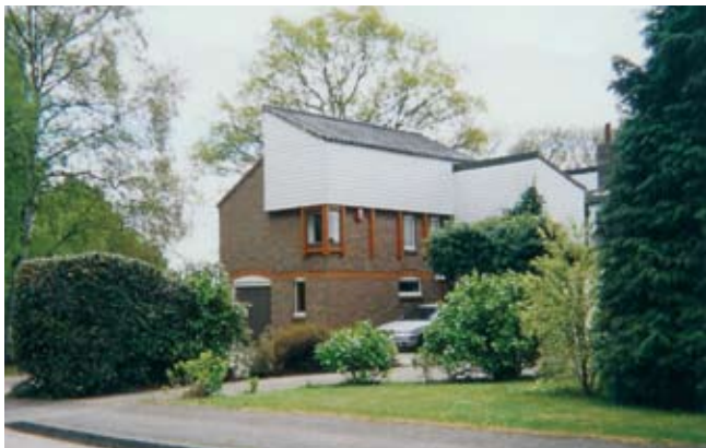
Modern styling - Hopping Jacks Lane
