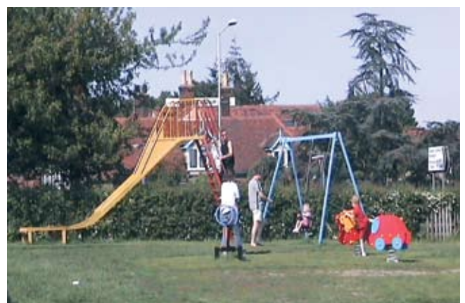
The environment of the children’s playground has been greatly improved by removal of the bark pits and installation of rubberised safety flooring
