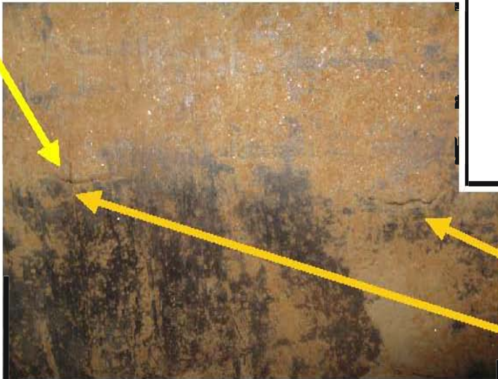
Figure 3-8: Interior View of Indentations Adjacent to Flange Section
