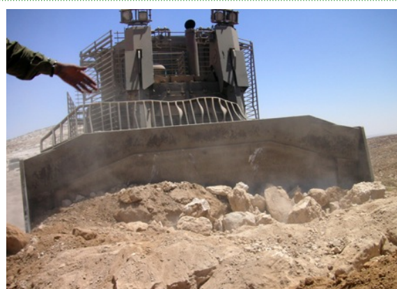
Israeli military bulldozer digging up Palestinian road near Jinba
