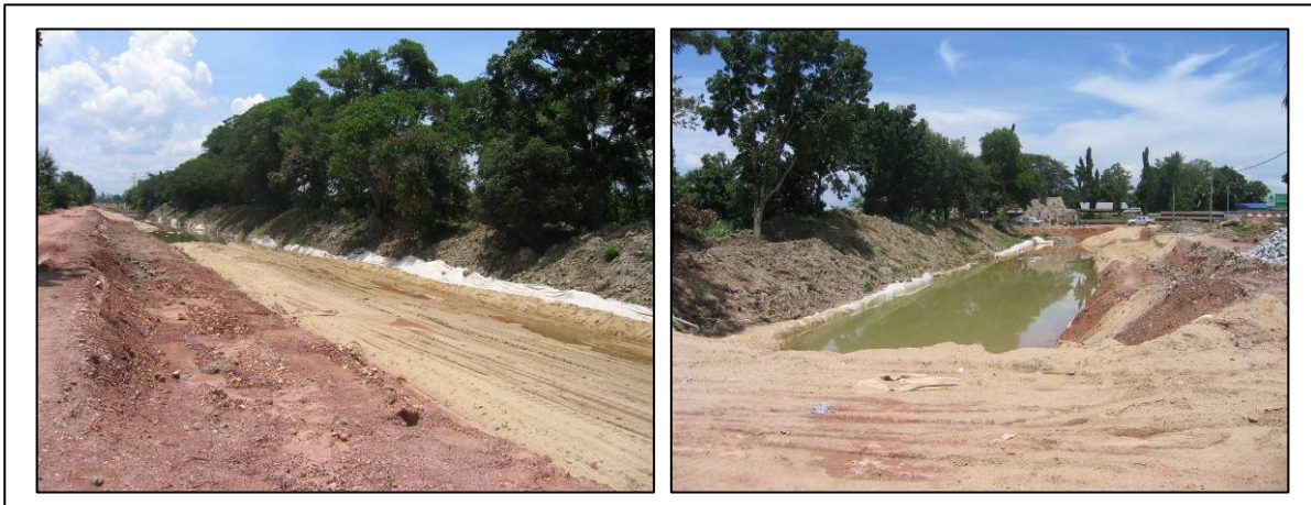
Figure 2.11 Construction Works at Pekula Pumping Station
