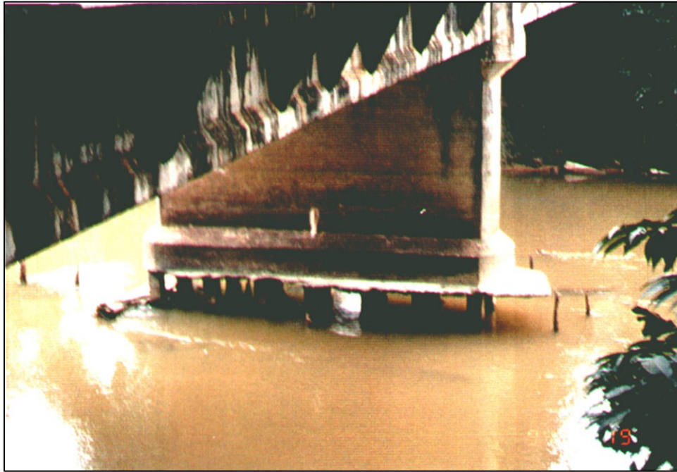
(1) Bridge Crossing Sg. Ketil (1km Upstream of Sg. Muda)
