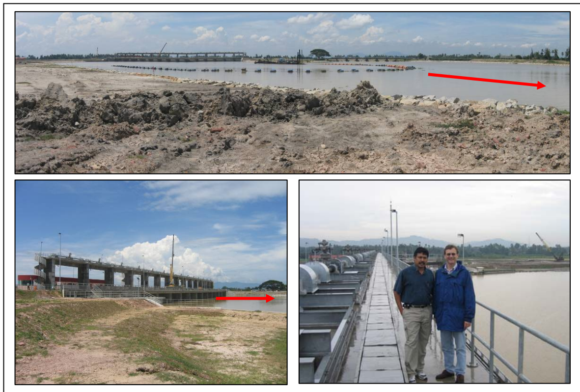
Figure 2.5 Construction of New Sg. Muda Barrage (CH 9400)
