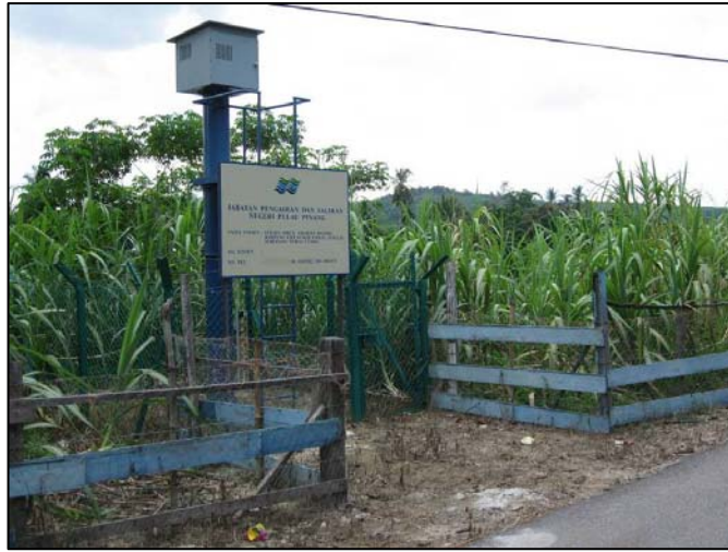
Figure 2.14 River Alarm Station @ Kampung Tepi Sungai Pinang Tunggal
