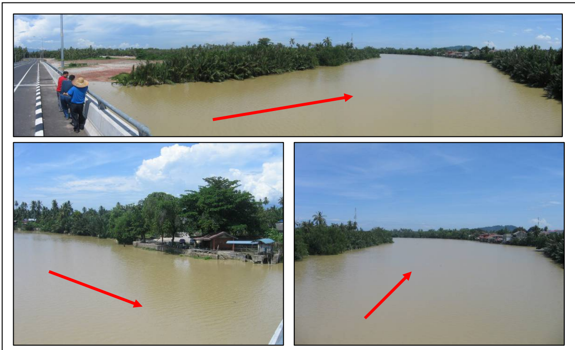
Figure 2.3 New Bridge at Sg. Muda Near Kota Kuala Muda
