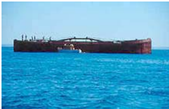
Preparing for demolition, April 1984
