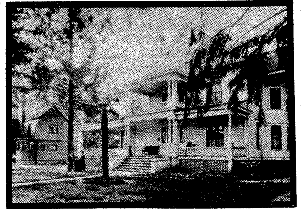
6. PATTERSON HOUSE: Built in 1903, at 751 East Eleventh Avenue, representative of fashionable homes built along the banks of the Millrace.
