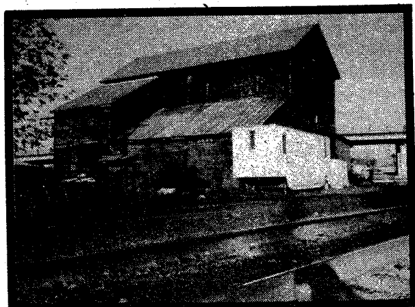
21. EUGENE MILL AND ELEVATOR COMPANY 1979: Only remaining Millrace industrial building located northeast of Fifth and High.
