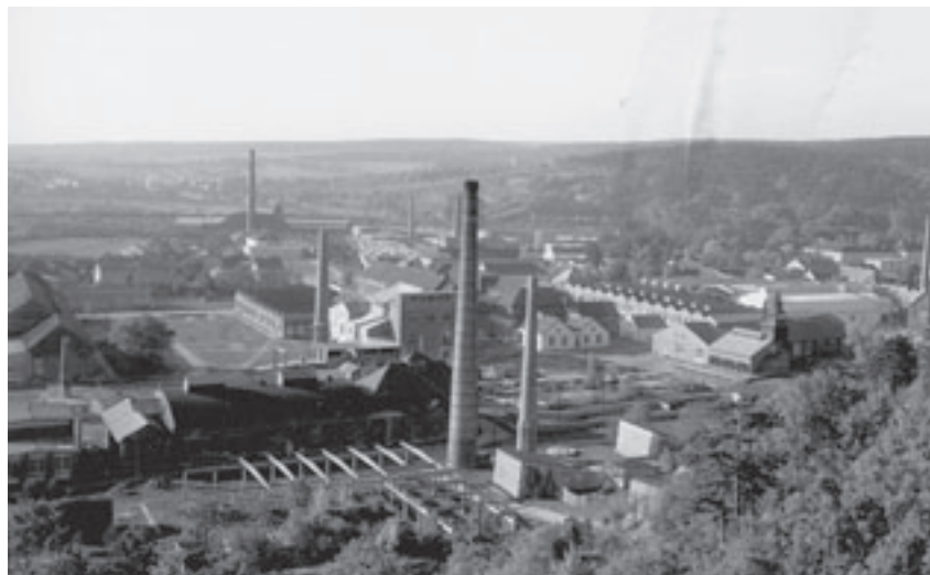
Ansicht des Talwerks, ca. 1955. / View of the Valley Works, approximately 1955.
