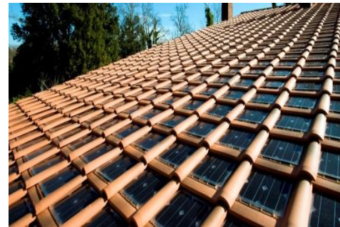
BIPV system with monocrystalline cells, 8 kW, Roma, Italy, courtesy of GSE
