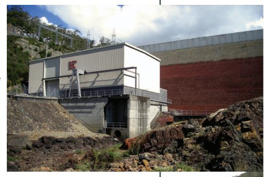
A riparian outlet pipe with regulating valve is installed to control water flow into the Forth River when the station is not operating.
