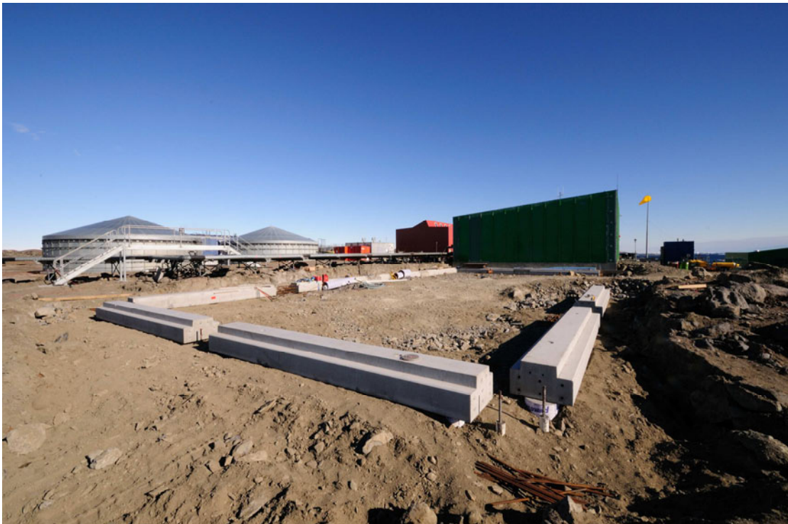
Figure 7.4: Pumphouse extension foundations
