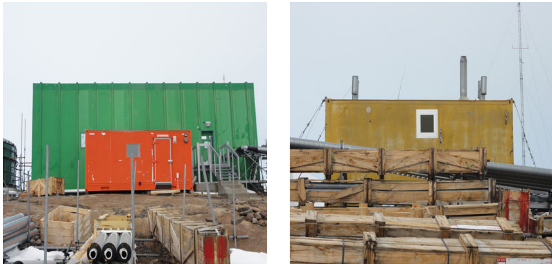
Figure 7.7: Site Service huts located near water holding tanks.
