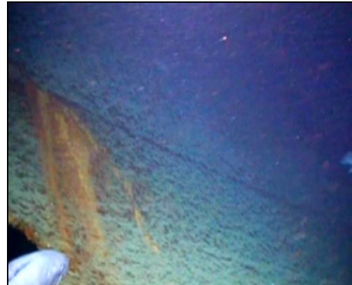
Figure 71: Rust around stern quarter area (Photo: DMS 2007)
