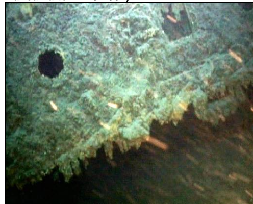
Figure 33: Starboard deck edge with scuttles and escape hatches, fairlead and rusticles (Photo: DMS 2007)
