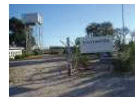
Namwater Purification Plant
