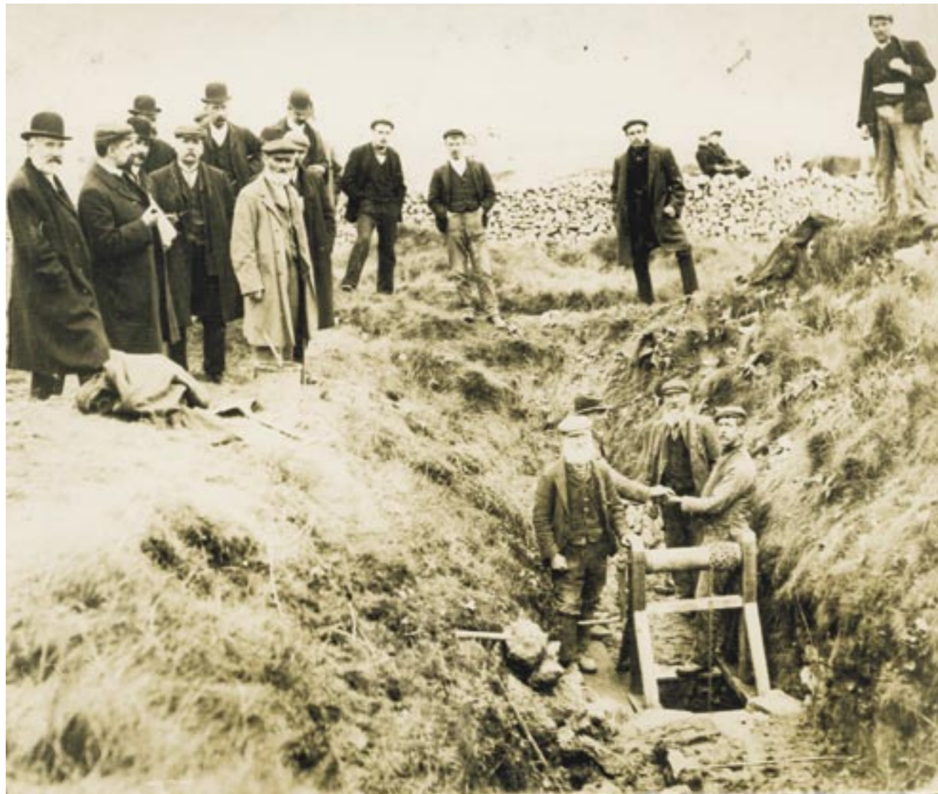
Mr Eagle, the King's Barmaster, handing over a disused lead mine on Moss Rake at Bradwell to a new group of miners in 1906. They stand next to a small shaft entrance with hand windlass (PDNPA collection).
