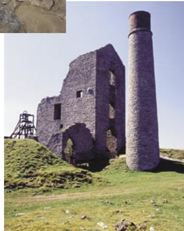
Magpie Mine near Sheldon has an exceptional surviving suite of buildings, including a 19th century Cornish engine house and chimney (centre/right) and a mid-20th century headgear (left) (photographer Jon Humble, English Heritage).
