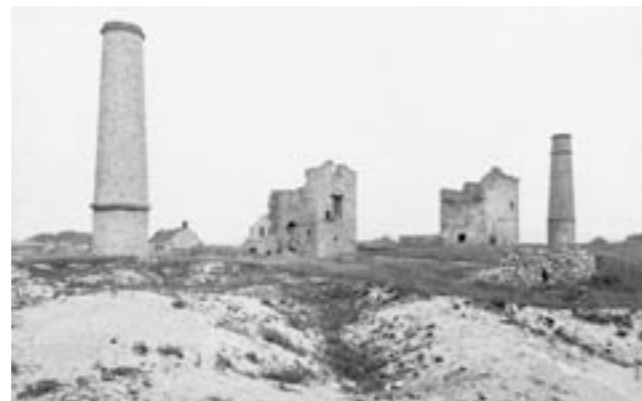
These impressive mine buildings at High Rake Mine near Great Hucklow were reduced to ground level in the 1920s. Their foundations are currently being excavated archaeologically by the Peak District Mines Historical Society conservation team (John Barnatt collection).
