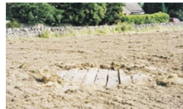
An impressive mining hillock at Elton (top) was recently removed after attempts to save it failed; all that remained afterwards were concrete sleepers sealing the mine shaft (PDNPA collection).
