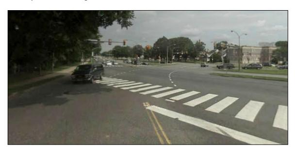
Existing sidewalk and crosswalk looking south at Adams Avenue are typical of the numerous diagonal roadway intersections which create hazardous crossings for pedestrians and, similarly, for bicyclists either in the road or on a sidepath. Although the Boulevard itself has three medians, some of the wider cross streets might be considered for bulb-outs or medians to break up the long crossings into manageable segments.
