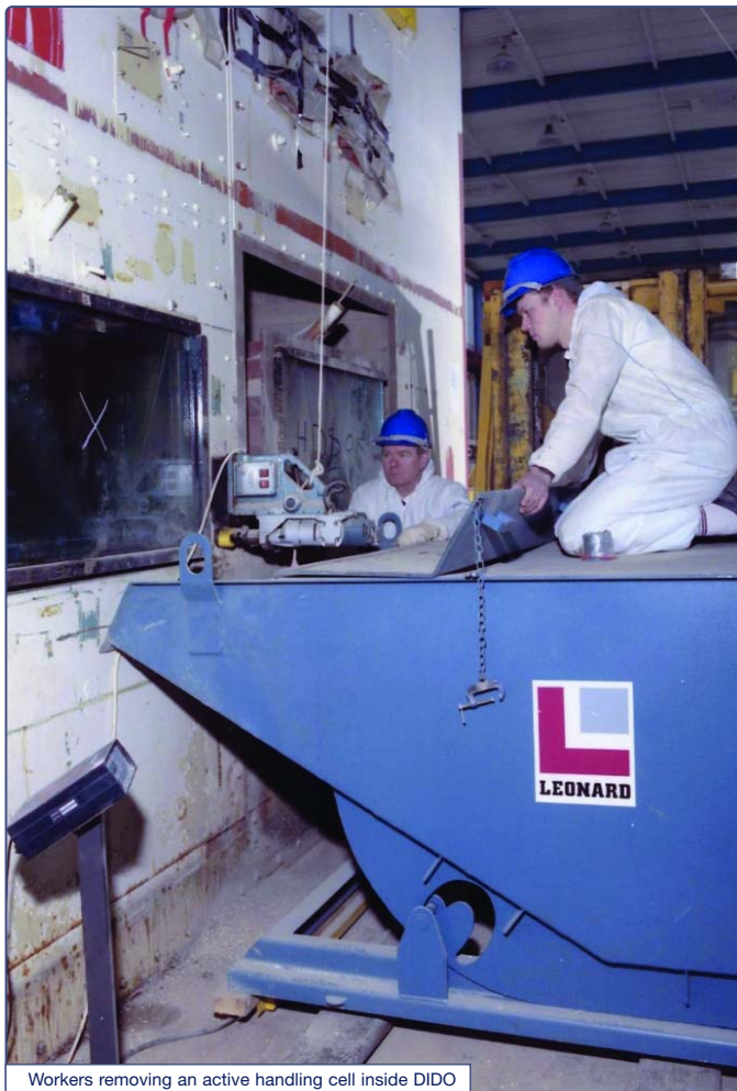
Workers removing an active handling cell inside DIDO
