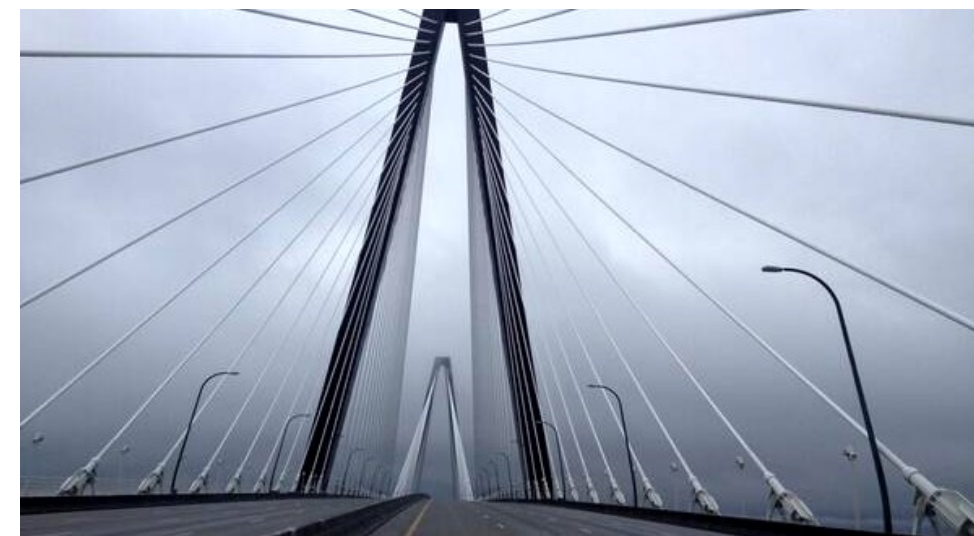
Closures to the Ravenel Bridge required re-routing Mt. Pleasant Services to the Don Holt.
