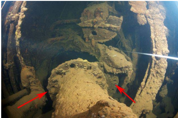
Flange E, left arrow: Flange E1, right arrow. Bulkhead at Frame 206 in background.
