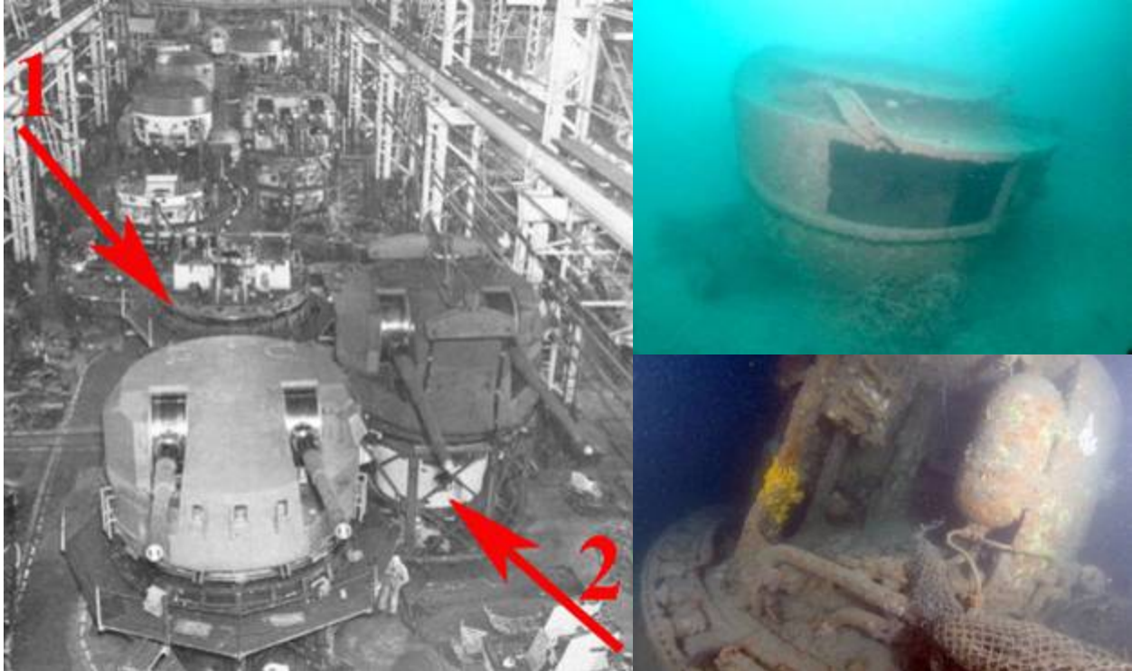
Left. Twin barreled 5.25-inch dual-purpose turrets under construction at the Vickers Armstrong facility. Note the incomplete turret's rotating roller ring in the background left (1) and the working chamber beneath the turret on right (2). For scale comparison note the man standing to the left of arrow 2. Top right. The inverted 'working chamber' on the seabed as seen if approached from astern. Bottom right. A close-up of the chamber, but as seen when approached from forward; note the 'roller ring' at bottom left.
