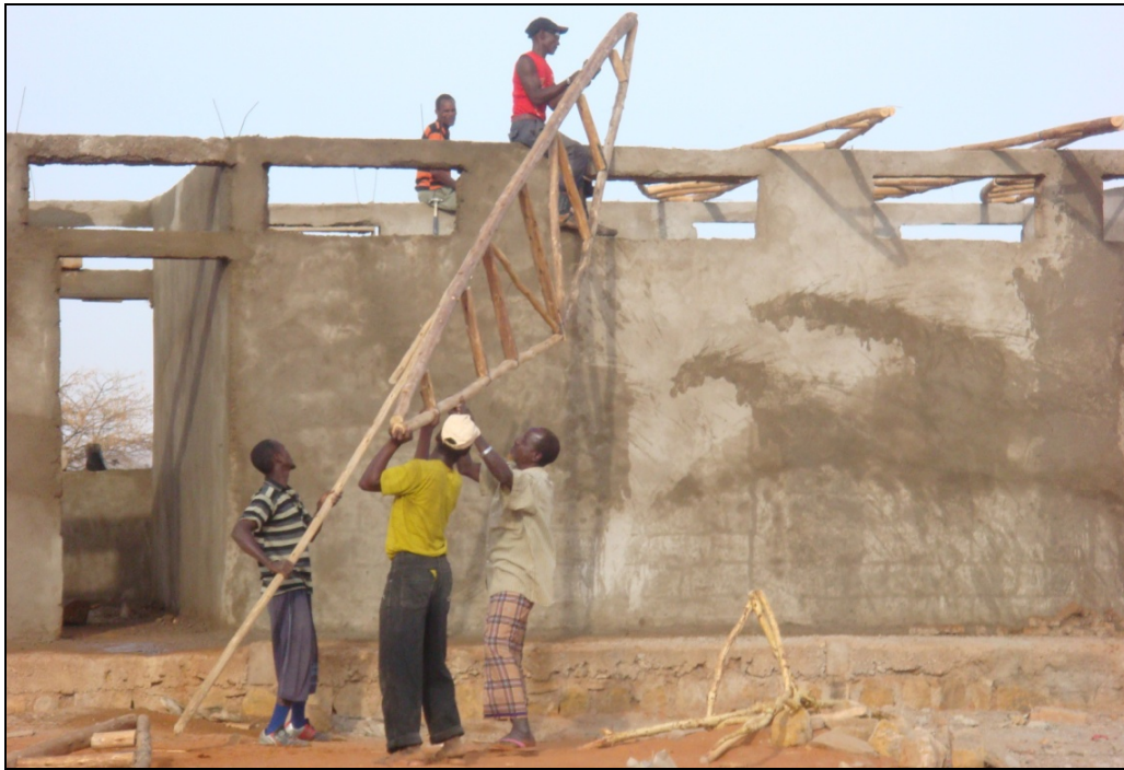
Construction of a new school in Hargelle woreda
