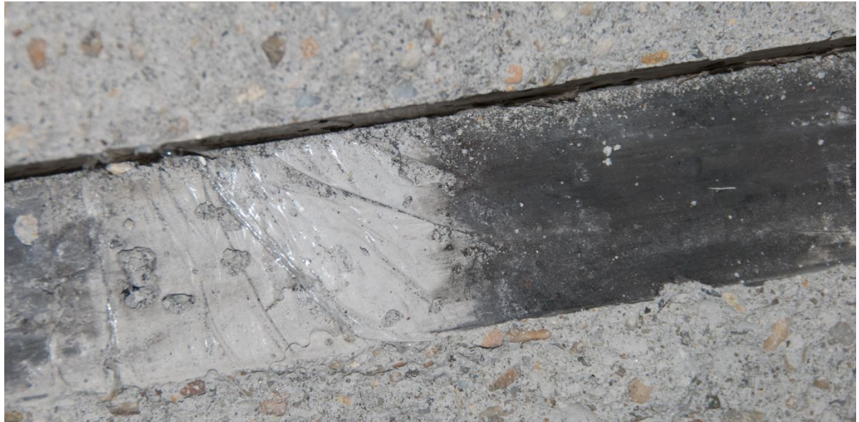
Figure 34 – Close-up view of the concrete surface shows no cracks or damage
