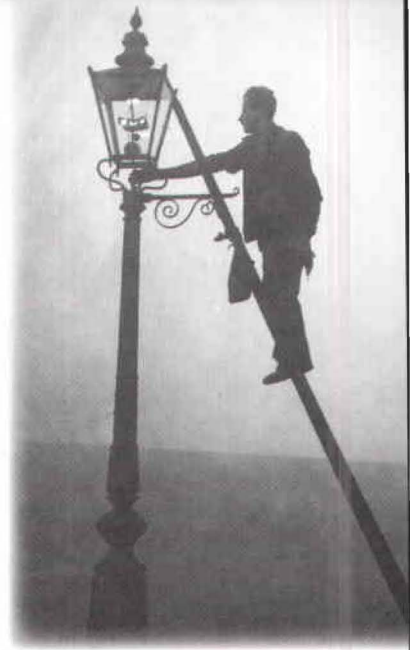
Gaslights were dangerous.
