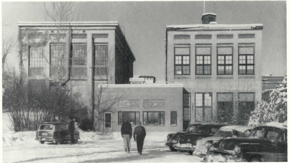
Above photo shows an overall view of the recently completed new addition and entrance to the Research and Development department building, Upper Main Street. Also shown is new parking area for Research employees and visitors.
