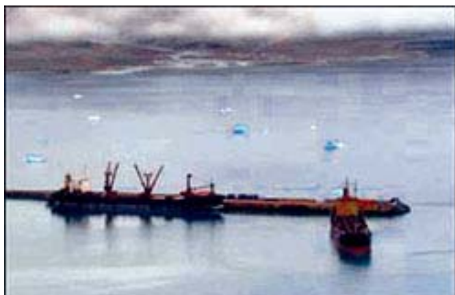
Thule Air Base Pier
