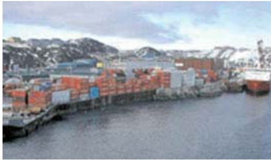
Nuuk (Godthab) Container Quay
