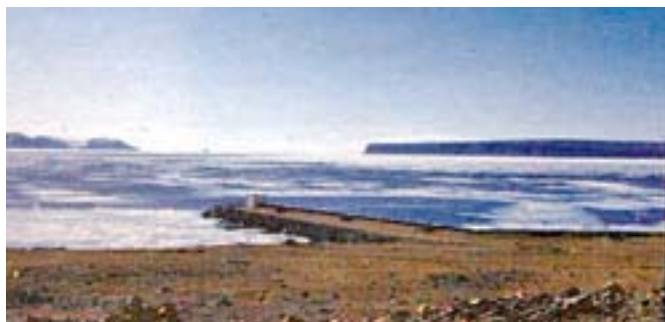
Thule Air Base Pier
