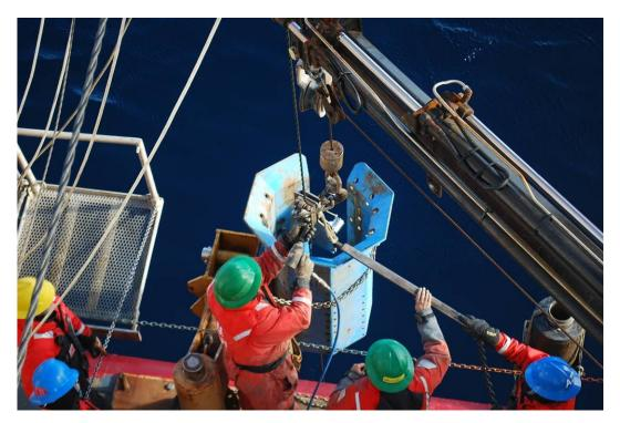
vii. Now you are ready to recover the jumbo piston core. Aframe boom out and take in wire slowly. Once the core appears, spot over the pivot stand. Using a 2x4, rotate
