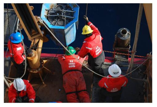
xi. Hook the crane block into the lifting point.<sup>1</sup> Slew outboard slightly and begin lifting the core barrel. As weight is taken, electrical tape holding the lifting wire to the
