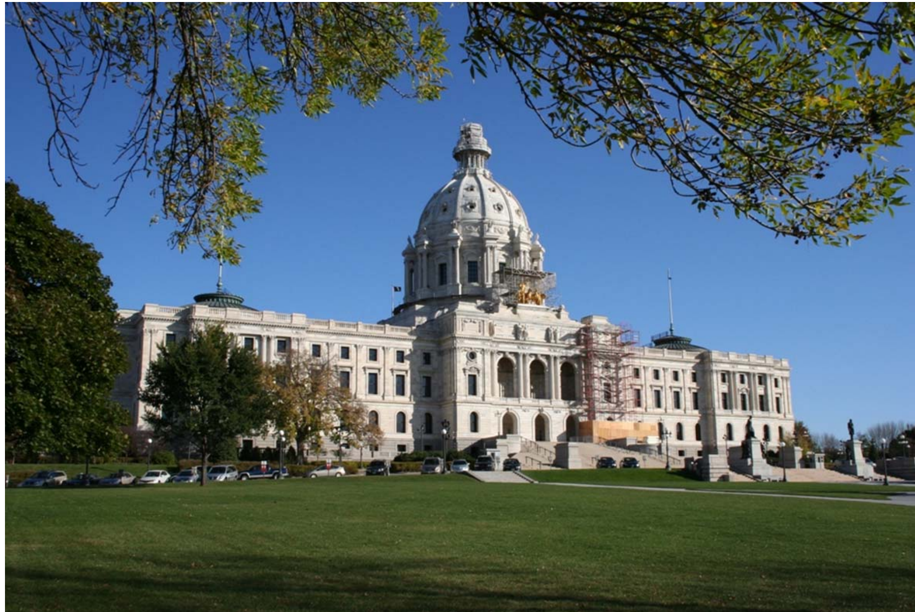
Existing Minnesota State Capitol Building 2011
