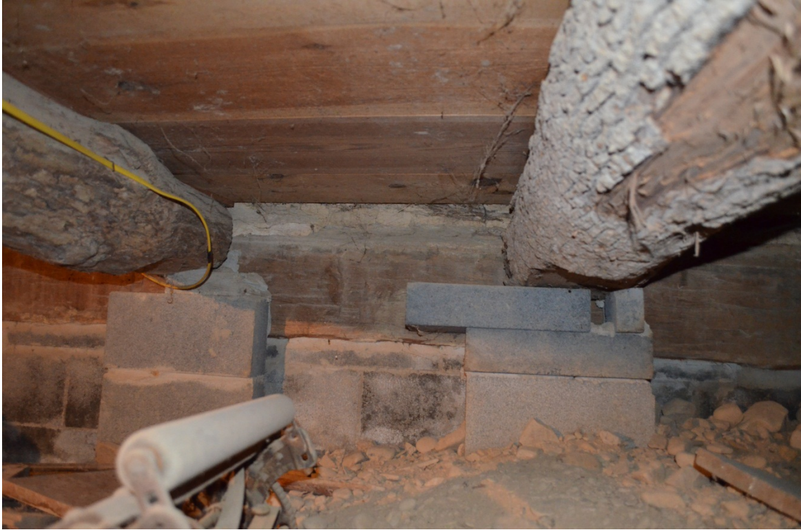
Photo 11: Detail of foundation piers, facing south
