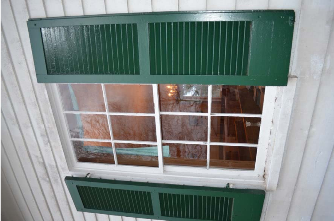
Photo 5: Detail of window, camera facing north
