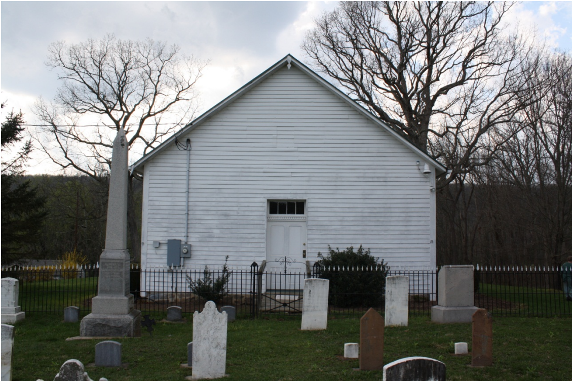
Photo 1: East elevation, camera facing west
