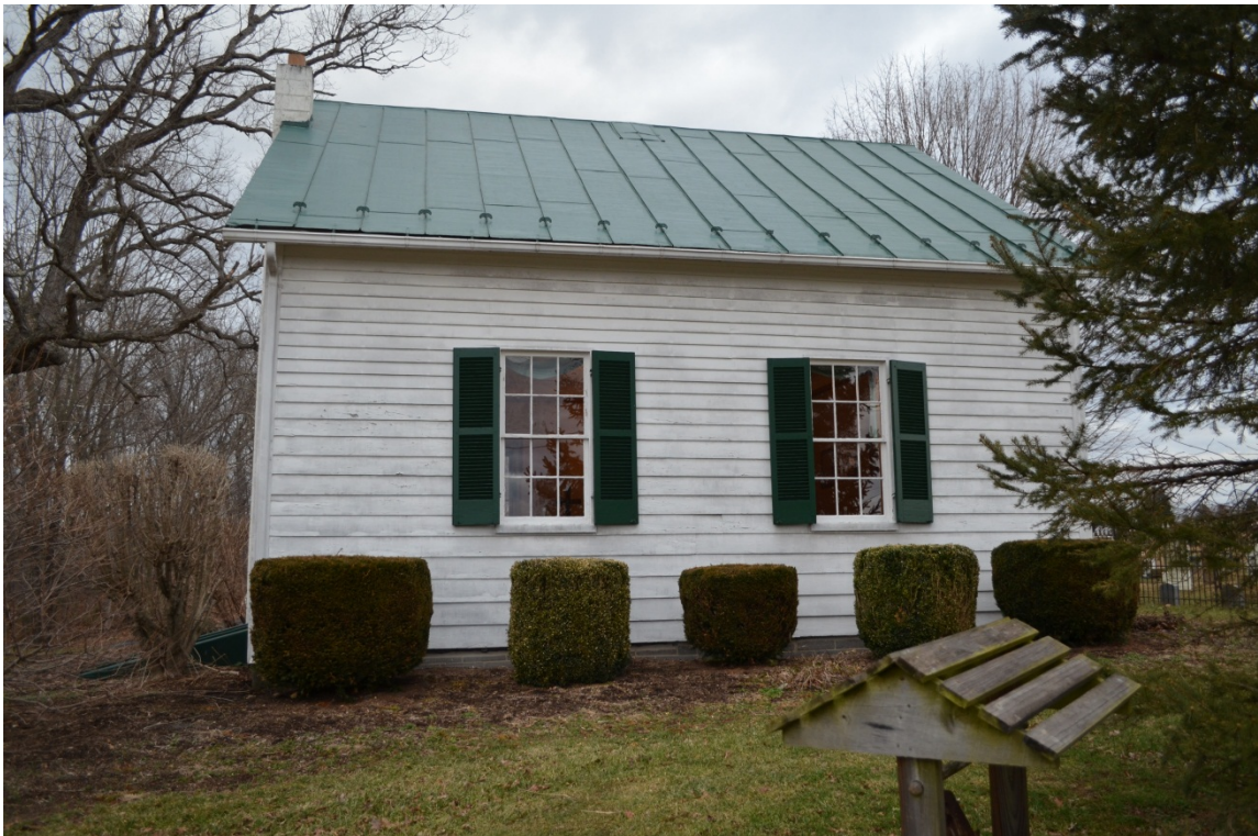
Photo 2: South elevation, camera facing north
