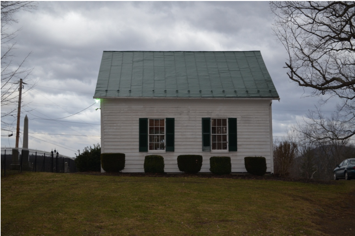
Photo 4: North elevation, camera facing south
