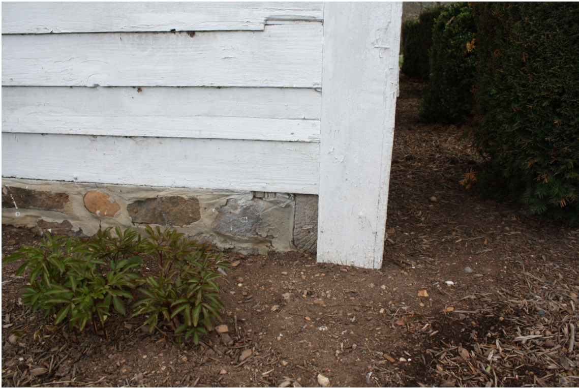
Photo 6: Detail of foundation, facing west
