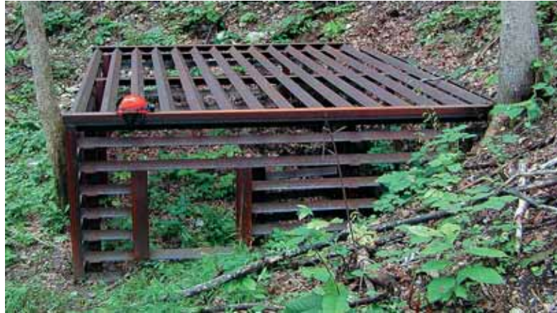
FIGURE 3 A cupola or cage style of cave gate allows bats to gain altitude and exit laterally, which is easier than flying up through a horizontal grate.
