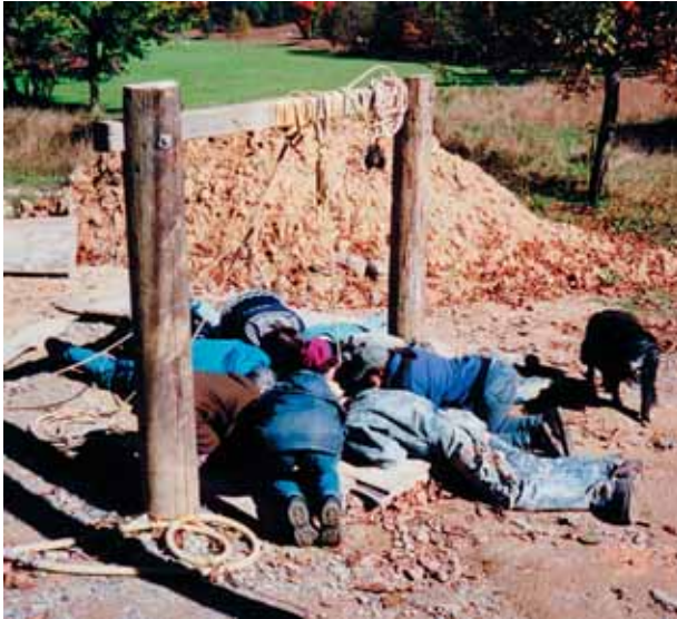
FIGURE 13 “Sidewalk superintendents” gather around Big Bucks Pit. The third entrance to Barberry Cave began as a drill hole followed by a 6-foot diameter shaft hand “dug” down to the top of the 80-foot high ceiling in the cave. In this photo, cavers are gathered around the top of the shaft, peering down to observe the “digging” activity at the bottom of the shaft.
