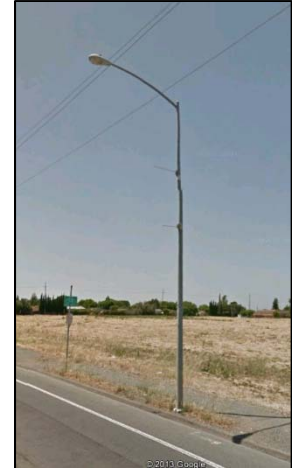
Figure 3-4: Typical CSA L-100 Street Light
