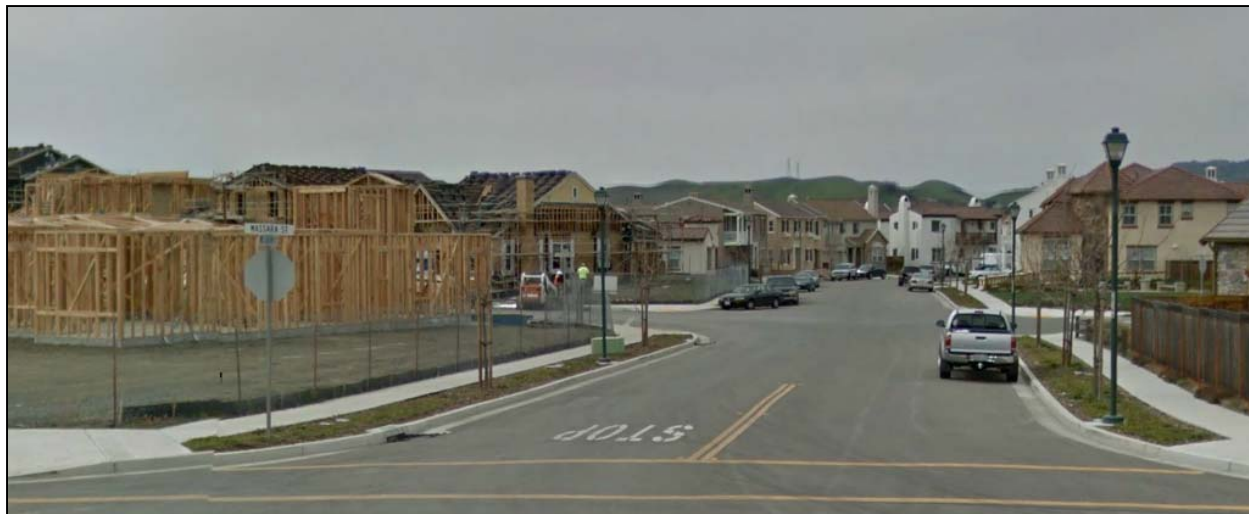
Figure 3-16: Housing Construction on Griffon Street, 2012
