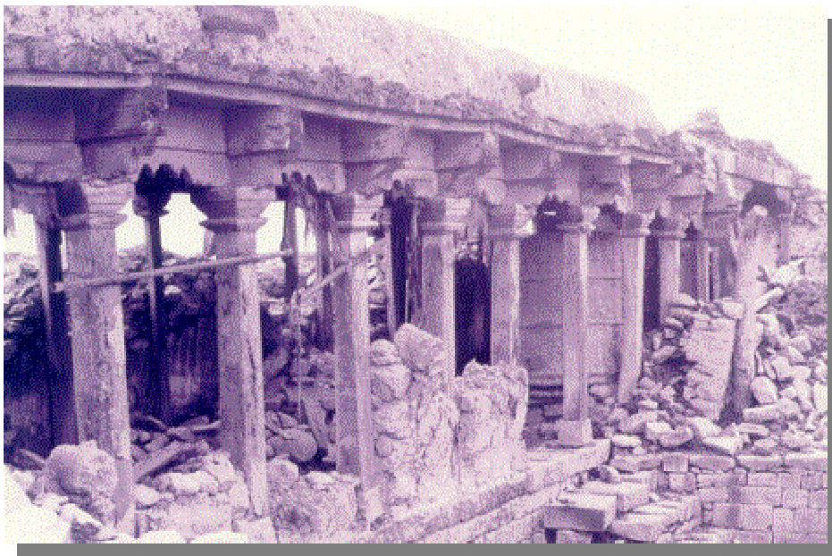
Figure 4: In some buildings, the traditional heavy clay roof was supported on a frame of wood posts and beams. In most cases, the timber columns continued to hold the roof together while the walls collapsed, generally outwards from the timber frame, saving the lives of many occupants
