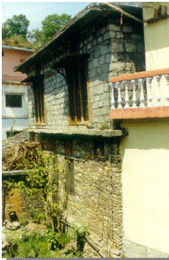
Figure 8: Partial collapse in a random rubble stone masonry. Note that the front portion has RC beam supported on concrete block columns and roof consists of RC slab
