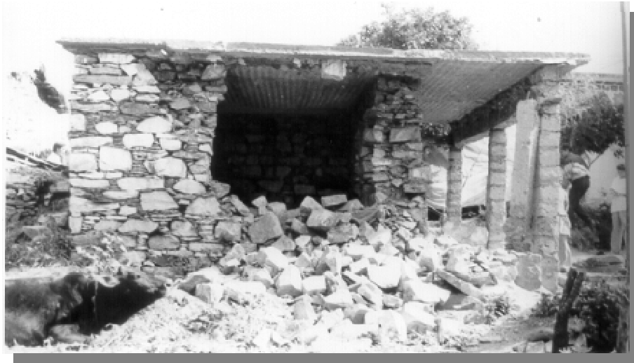
Figure 8: Partial collapse in a random rubble stone masonry. Note that the front portion has RC beam supported on concrete block columns and roof consists of RC slab
