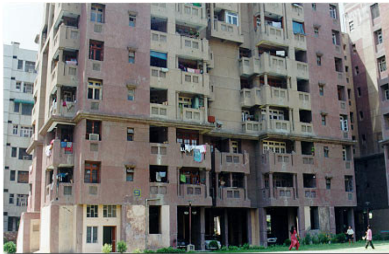
P3. Tarang Apartment in Delhi that sustained damage to infill walls.
