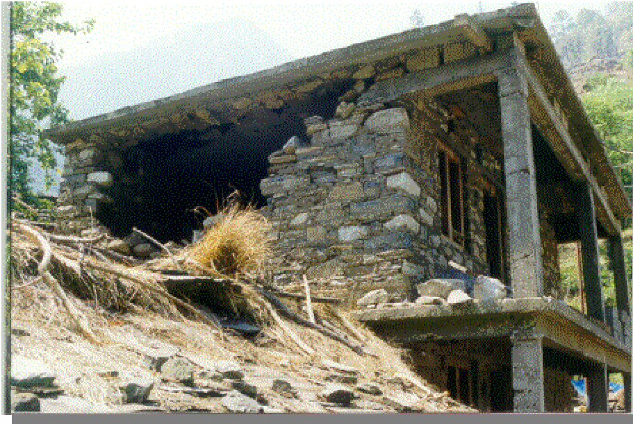
Figure 10: Partial collapse in a stone masonry house at Gadi village. Lintel band, present in the front portion, does not continue in the side wall
