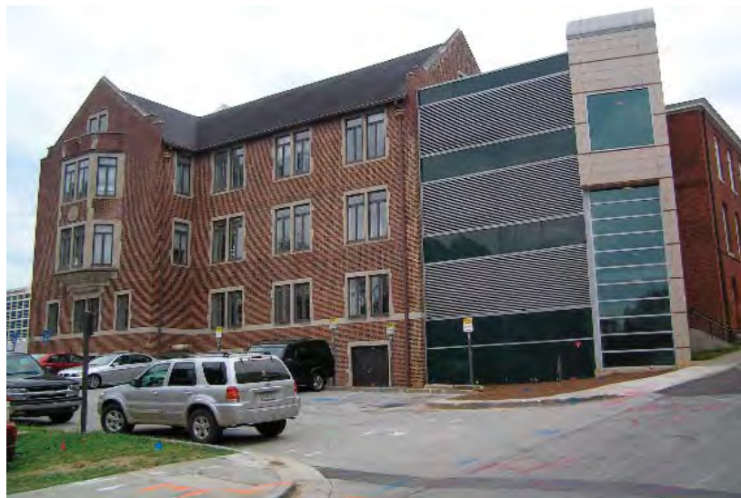
View of William Henry Emerson Building looking south.
