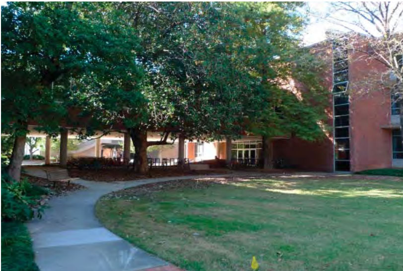
View of the courtyard at the Architecture Building (East) looking northwest.
