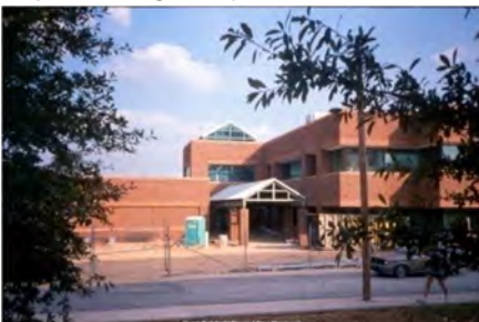
Figure 94: 1988 view of the Joseph M. Pettit Microelectronics Research Building (Image from Georgia Tech Capital Planning & Space Management)
