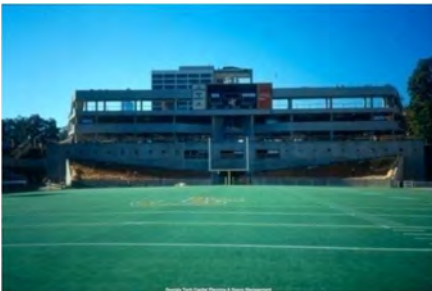
Figure 93: 1987 view of the William C. Wardlaw Jr. Center under construction (Image from Georgia Tech Capital Planning & Space Management)
