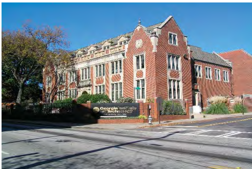
View of Daniel F. Guggenheim Building looking northwest.
