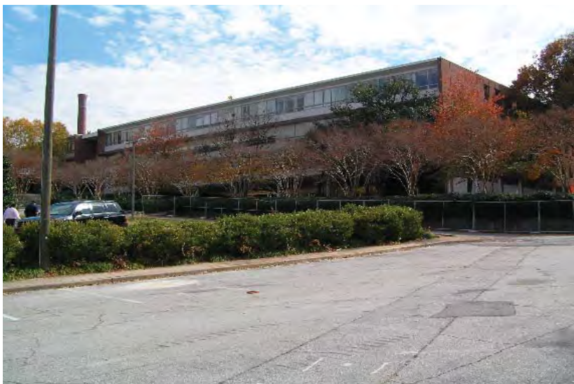
View of William Vernon Skiles Classroom Building looking south.
