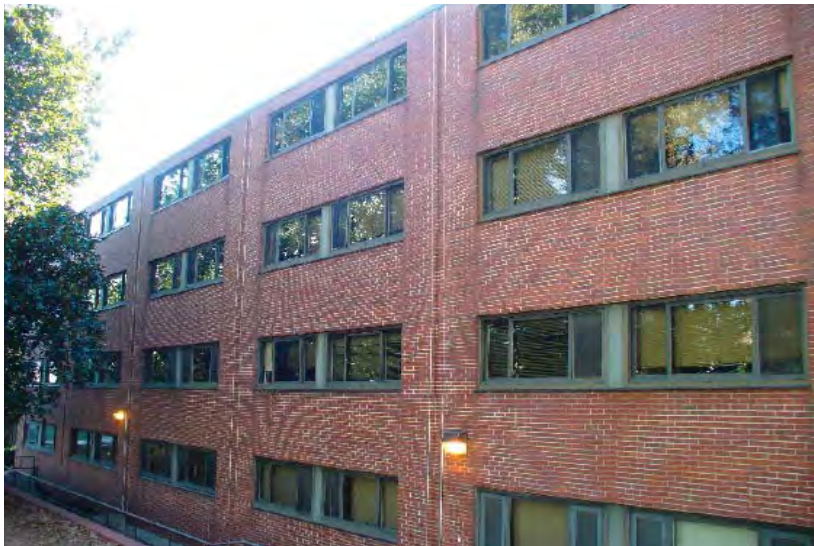
View of typical elevation of the Major John Hanson Residence Hall.
