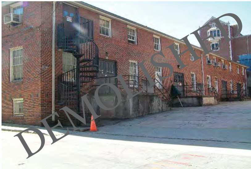
View of 220 Bobby Dodd Way (former Army Offices)
