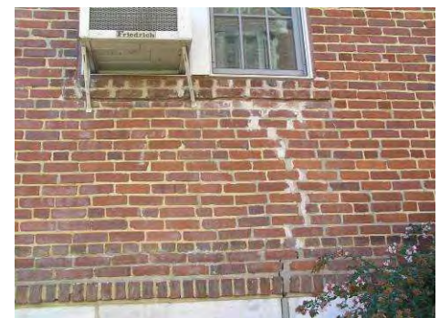
Figure 107: The repointing of mortar joints should use mortar that is materially compatible with the historic masonry and should also be visually consistent with the adjacent work.
