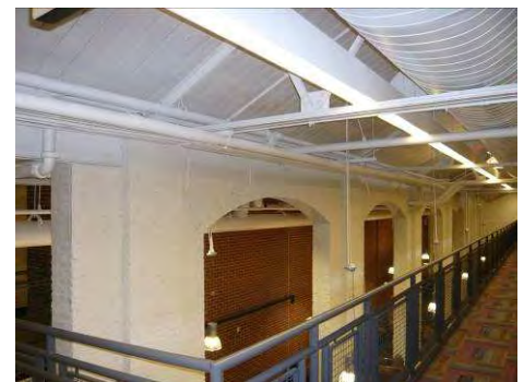
Figure 110: The historic masonry walls and arched openings have been integrated into this interior rehabilitation of the John Saylor Coon Building.
