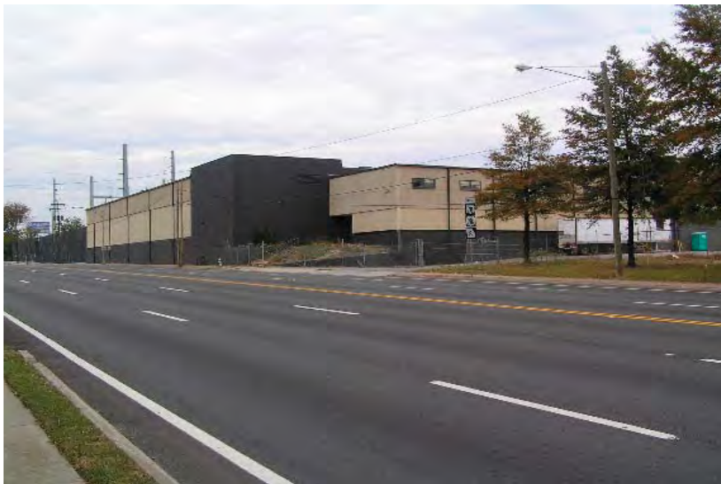
View of 645 Northside Drive, N.W.
