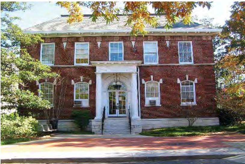
View of Lloyd W. Chapin Building looking east.
