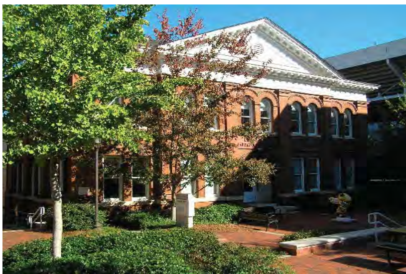
View of Lyman Hall Building looking northeast.
