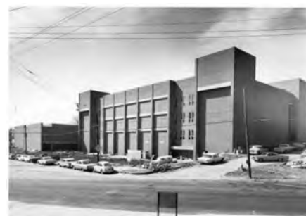
Figure 91: 1970 view of the Boggs Chemistry Building (Image from the Georgia Tech Capital Planning & Space Management)
