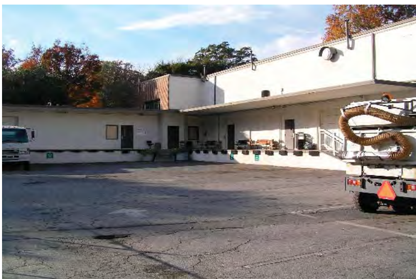
View of Facilities Garage/Warehouse looking northwest.
