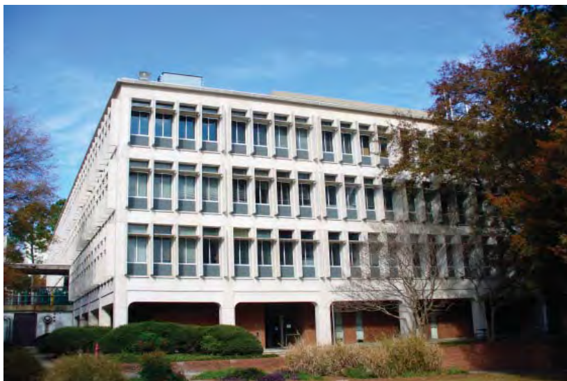
View of Bunger-Henry Building
