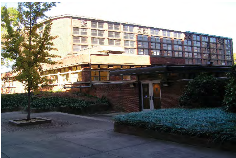
View of Hinman Highbay looking southeast.
