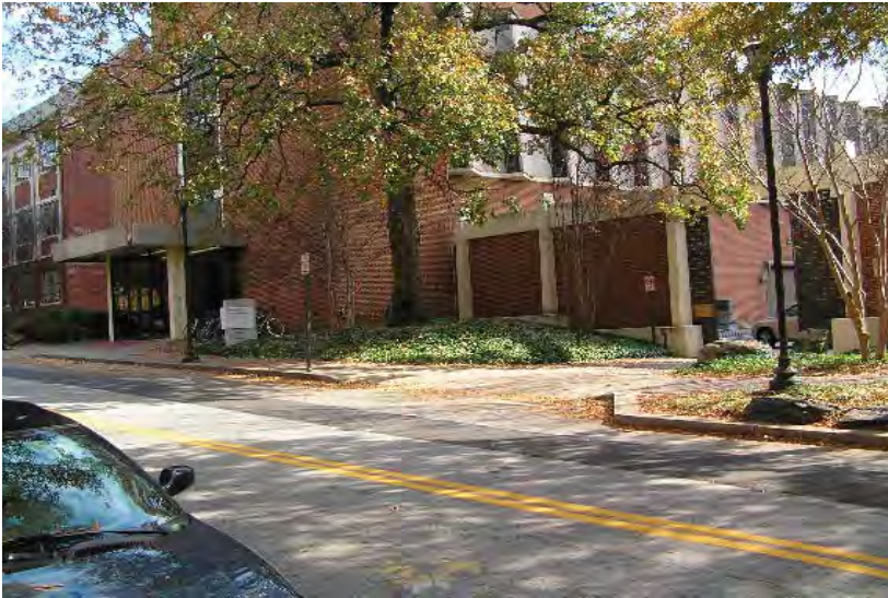
View of Montgomery Knight Building looking southeast.
