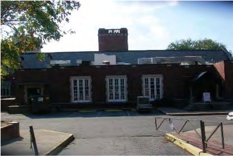
View of Marion L. Brittain "T" Room Addition
