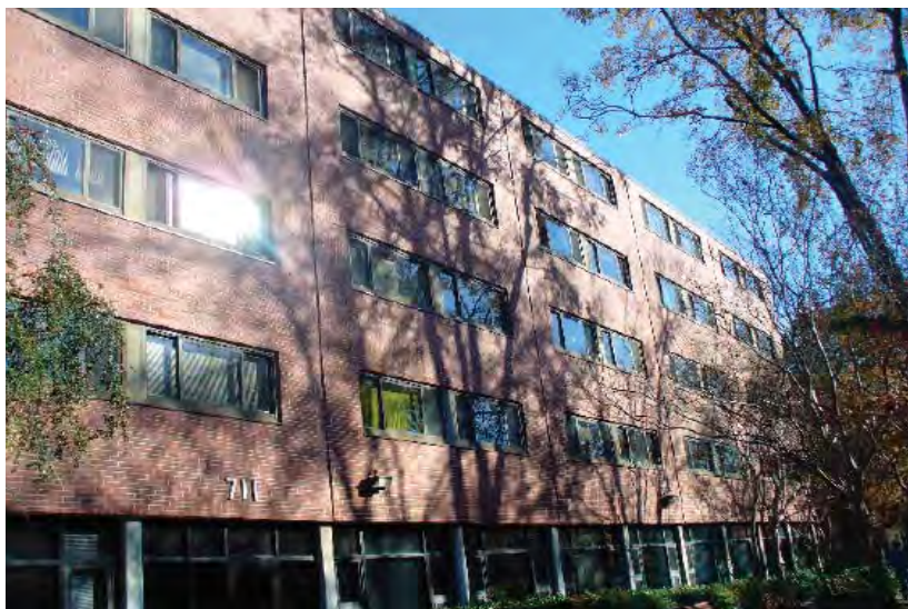
View of Floyd Residence Hall.
