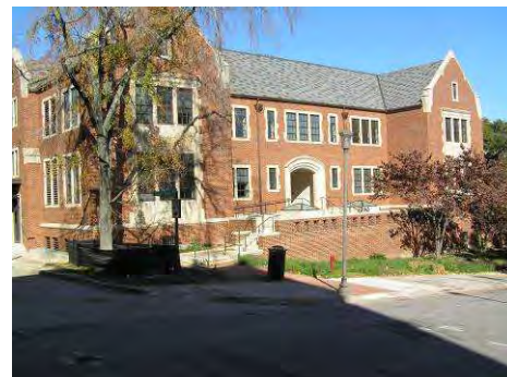
Figure 101: View of the recently rehabilitated Old Civil Engineering Building.
