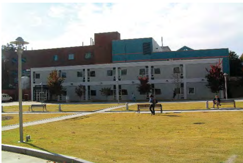
View of Architectural Annex Building looking west.
