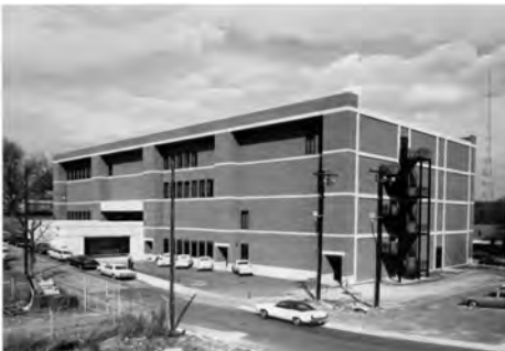
Figure 90: 1970 view of the Harry L. Baker Building (Image from Georgia Tech Capital Planning & Space Management)
