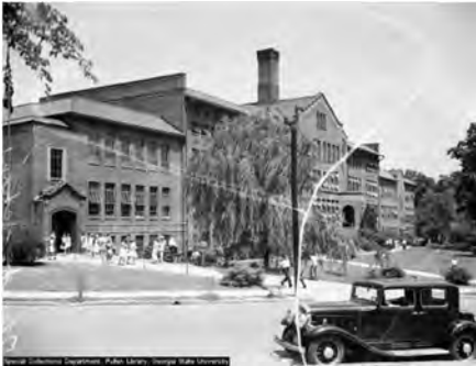
Figure 68: 1949 view of the Daniel C. O’Keefe building (Image from Special Collections Department, Pullen Library, Georgia State University)
