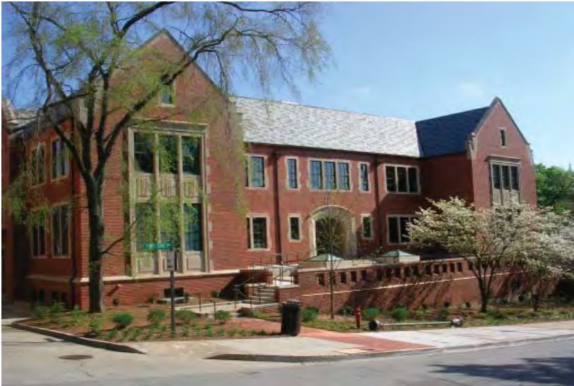
View of Civil Engineering Building looking northeast.
