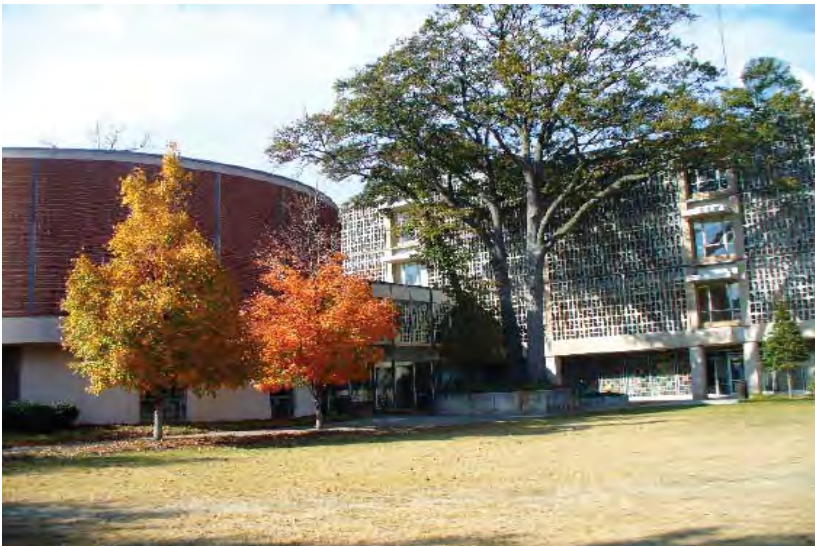
View of Blake Van Leer Building looking northwest.
