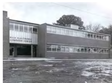
Figure 92: Early view of the Rich Computer Building (Image from Georgia Tech Capital Planning & Space Management)
