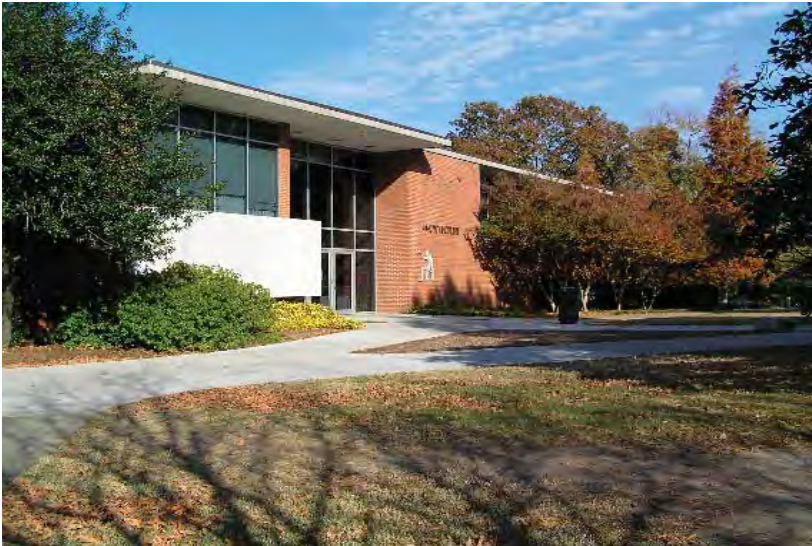
View of Architectural Building looking northeast.
