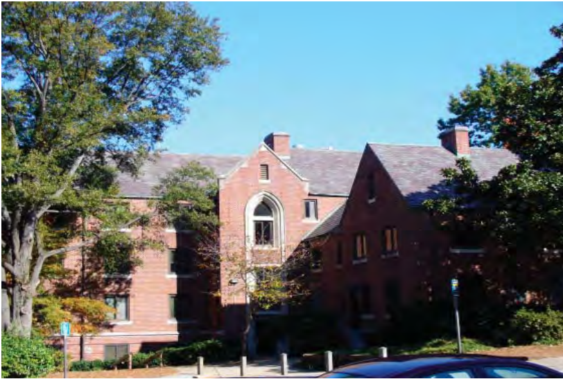
View of John M. Smith Residence Hall looking east.
