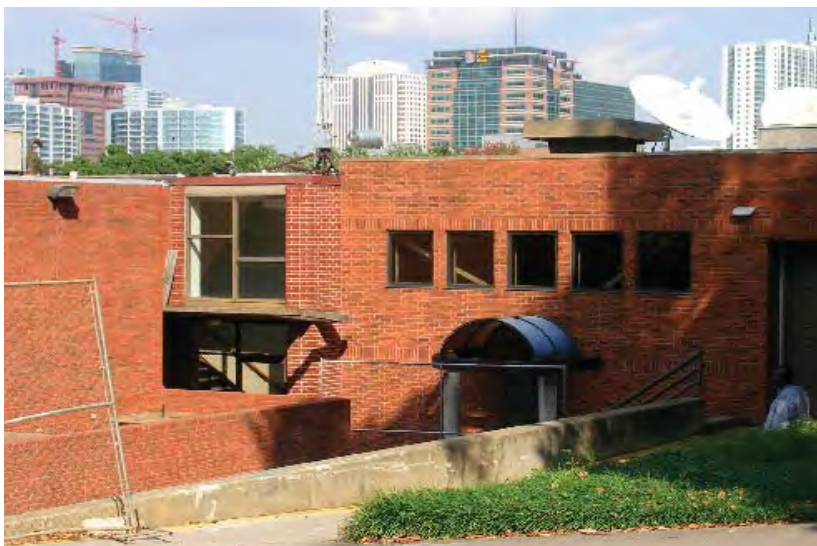
View of Rich Building looking southwest.
