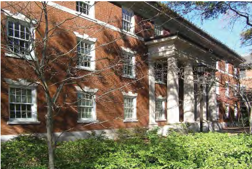
View of the Janie Austell Swann Building.
