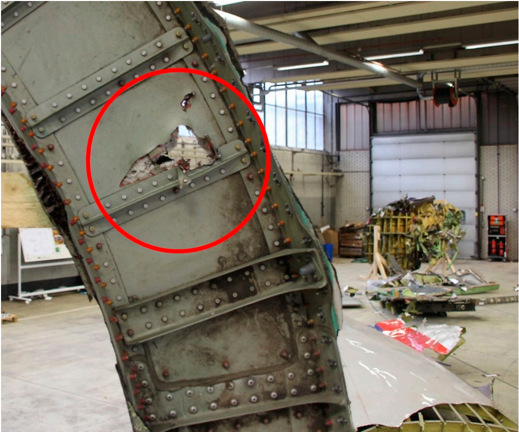
Figure 29: Impact damage on rear side engine cowling ring
