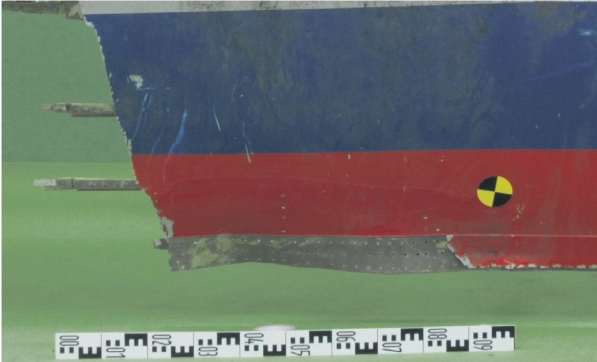
Figure 23: Typical case of longitudinal joint failure by peeling, in the right part of the figure. (Source: Dutch Safety Board)
