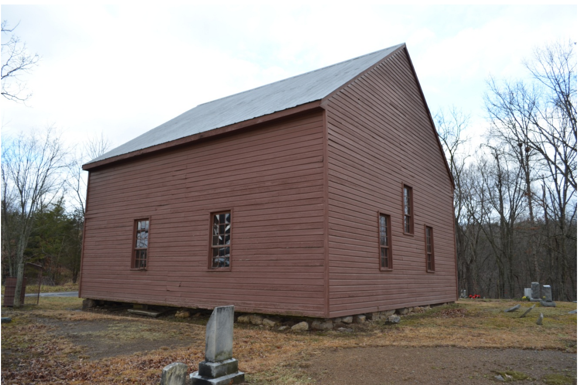
Photo 4: South and East Elevations, Camera Facing Northwest
