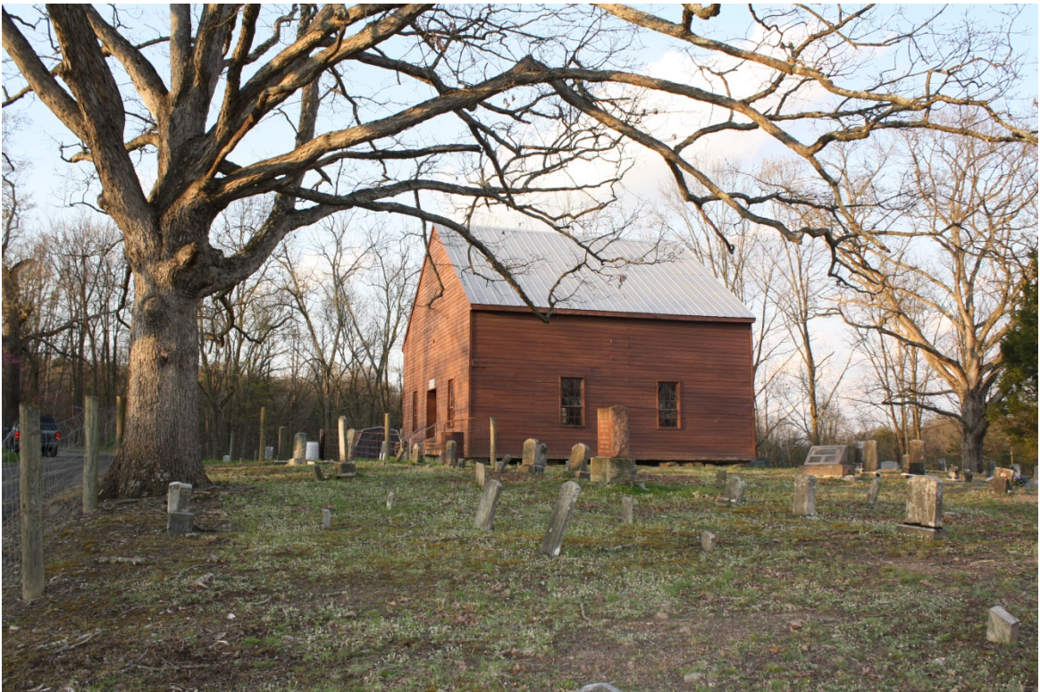
Photo 8: Old Pine Church, Facing Northeast
