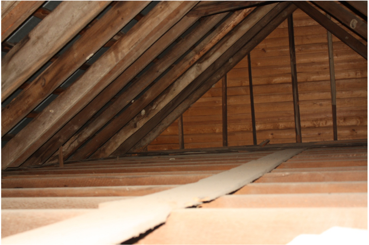
Photo 17: Interior of Attic Space, Facing East
