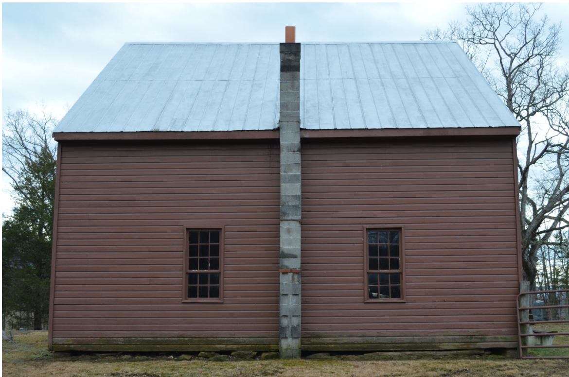
Photo 2: North Elevation of Old Pine Church, Camera Facing South
