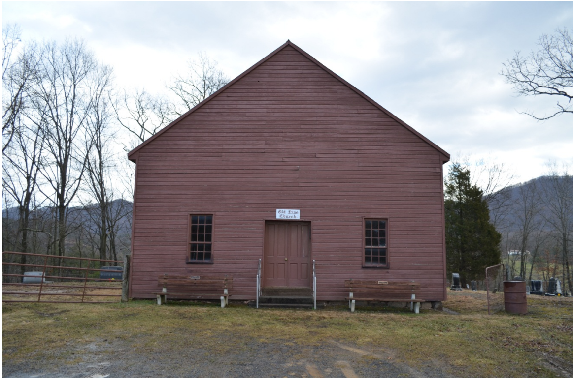
Photo 1: West Elevation of Old Pine Church, Camera Facing East
