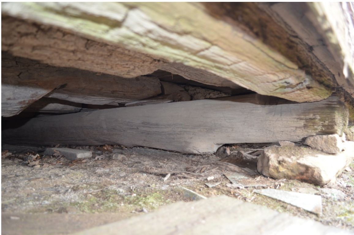
Photo 16: Foundation Detail Consisting of Stone Piers, Facing North
