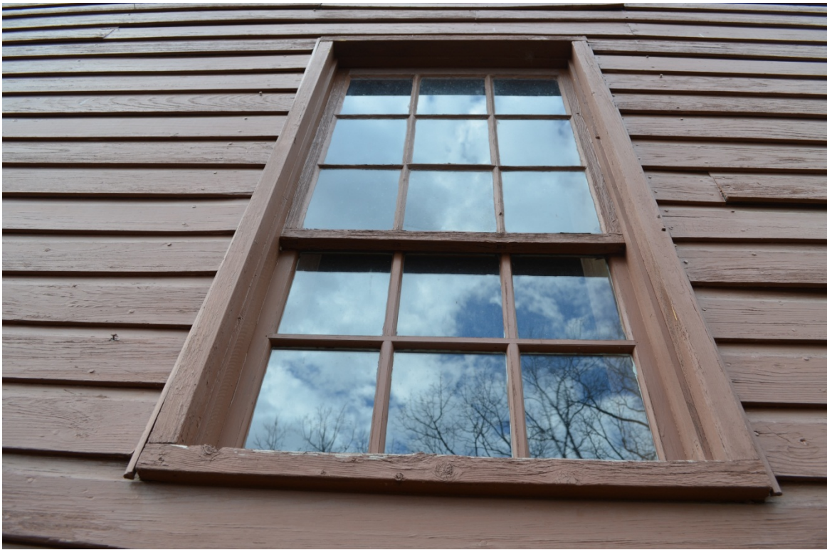
Photo 11: Detail of Window, East Elevation, Facing West
